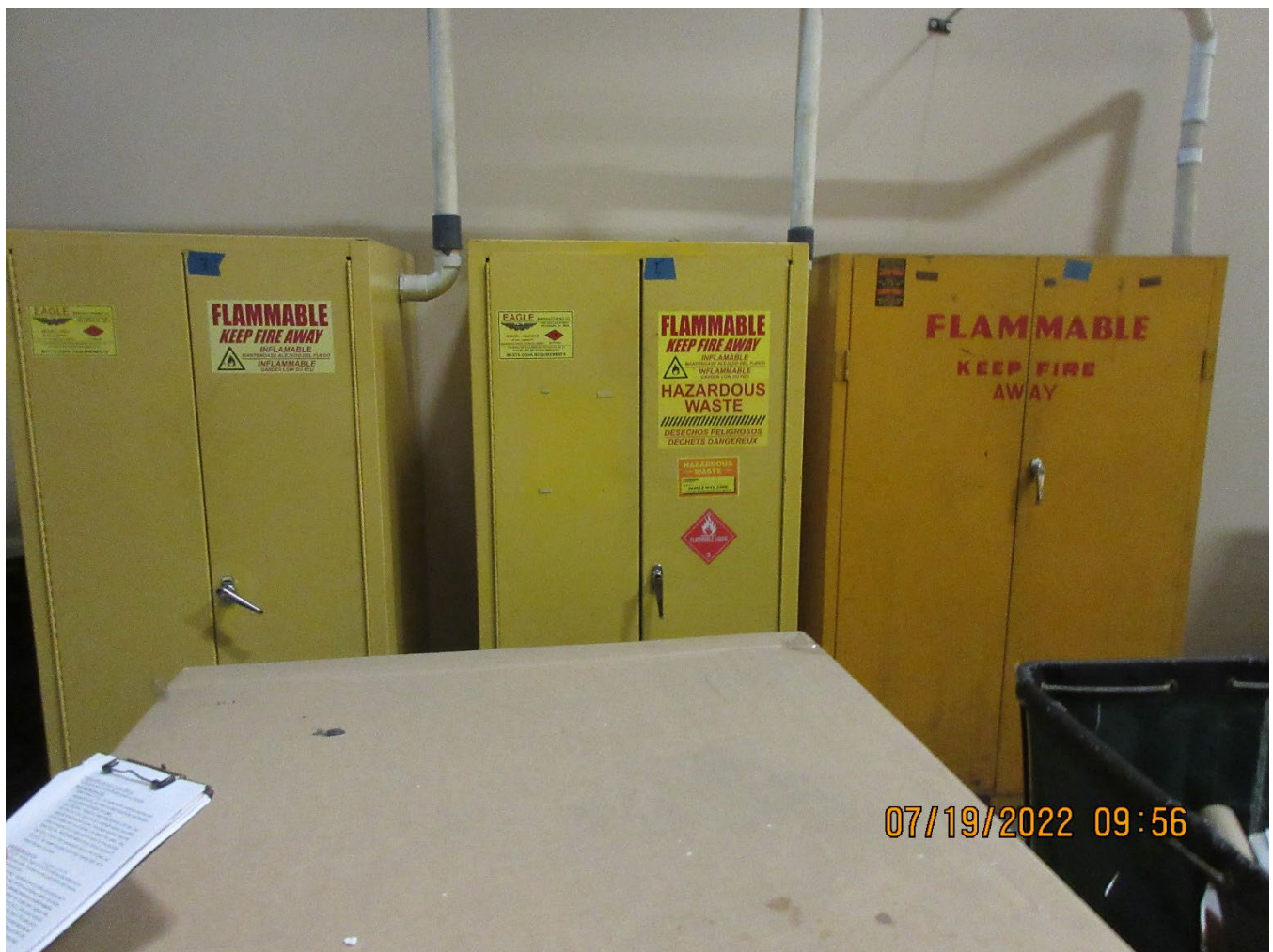
Photo 1 – Quality Control 90-Day Accumulation Locker (Center)
