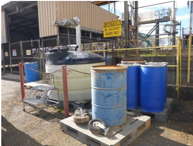
Photo 9: Two 55-gallon steel containers and three 55-gallon plastic containers on wooden pallets next to the used oil tank.
