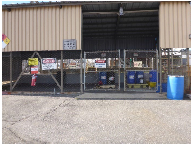
Photo 7: The Permitted Container Storage Area.
