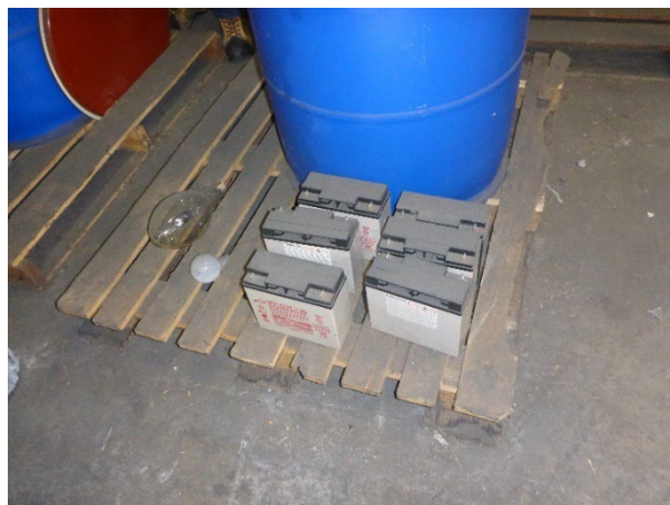
Photo 5: Six lead-acid batteries and one HID lamp on a wooden pallet at the Warehouse #3 CAA.
