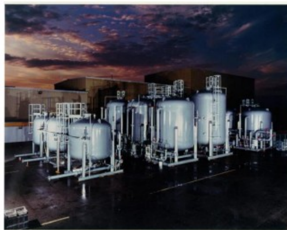
Figure 4: Tanks at the Manufacturing Plant.
