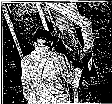
Applying J-M Type B batts in new home
