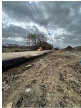
East silt fence replacement, per your photo where there was damage from the neighboring contractor.
