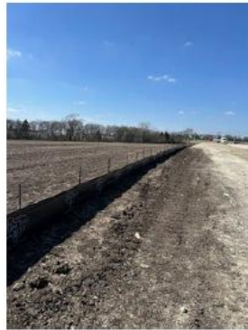
This is the area south extremity of the property where you saw we were grading the slope and behind curb.
