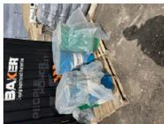
Curing compound barrels off the ground and covered.
