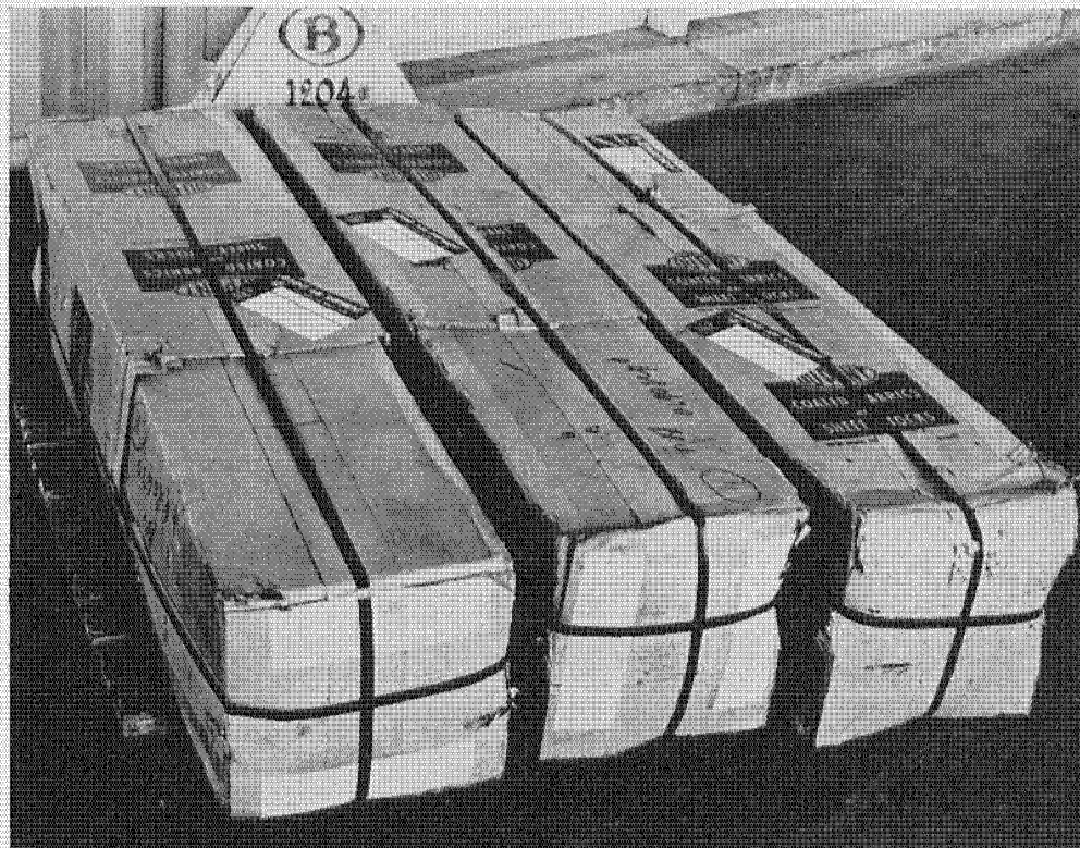
Photographed in Belgium after 3,000-mile trip, these containers of fabrics were battered and had telescoped. Resilient "Dymax" strapping, however, remained tight, still fitted snugly over cartons.
