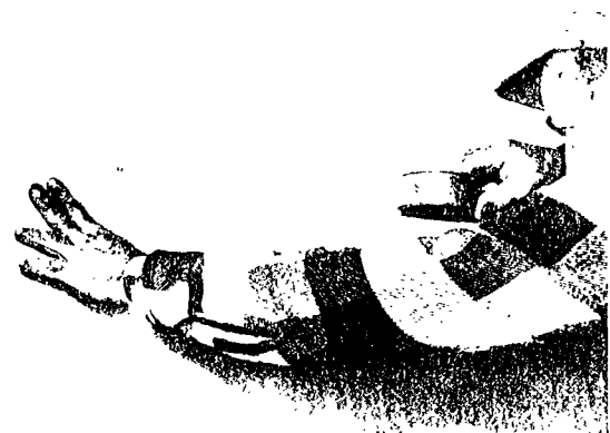
Apply Vinyl Tape to all joints where tile will be used. Use regular joint system above tile area.
