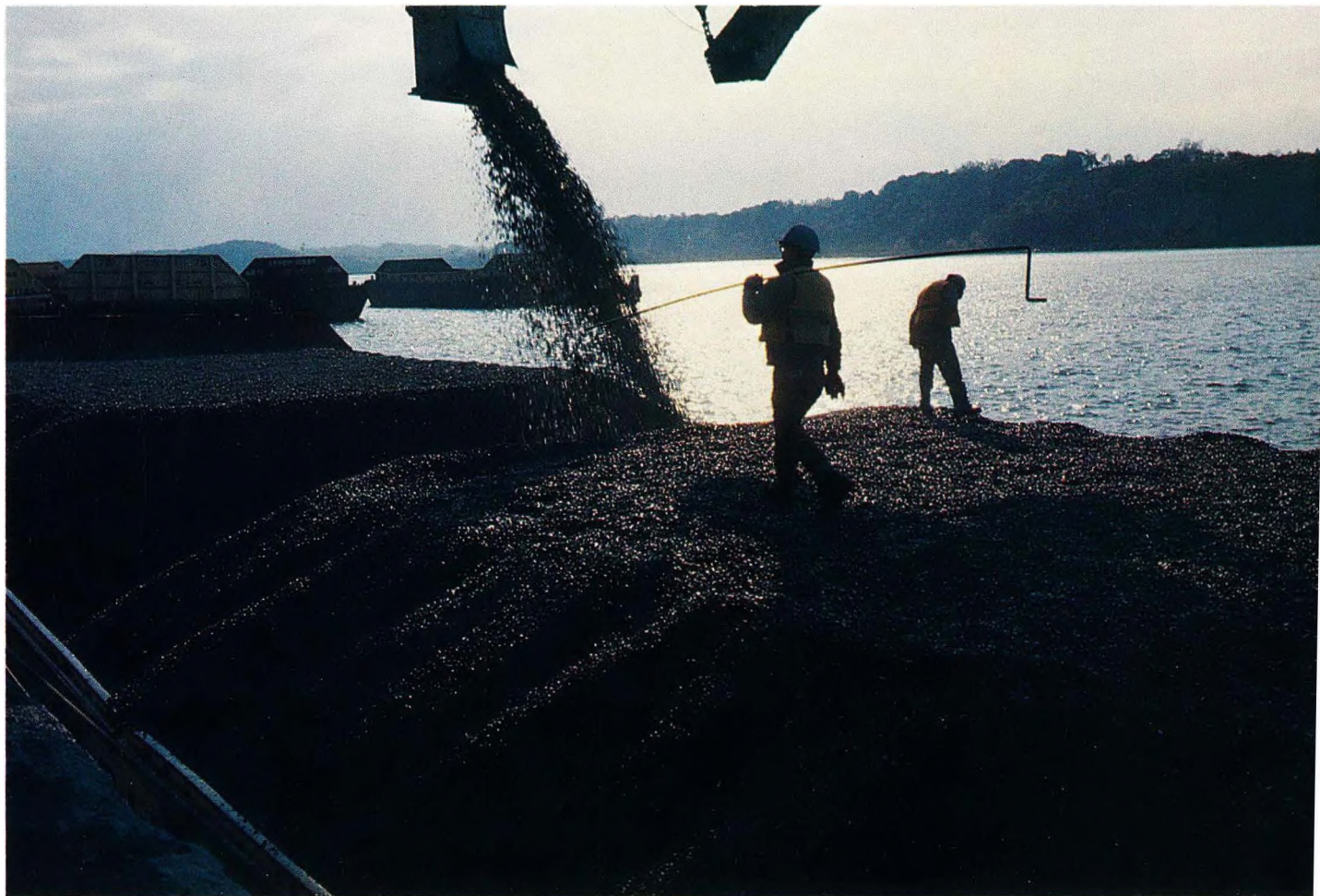
Above: Loading barges at Clinton Point, near Poughkeepsie, N.Y.
