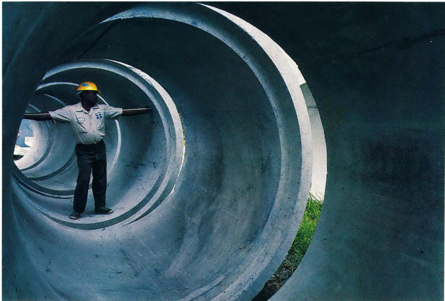
Above: Concrete mains precast at Charleston, S. C.
