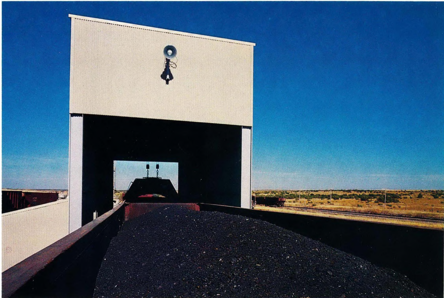
Preheaters (left) and coal-handling facility (above) at Maryneal, Texas
