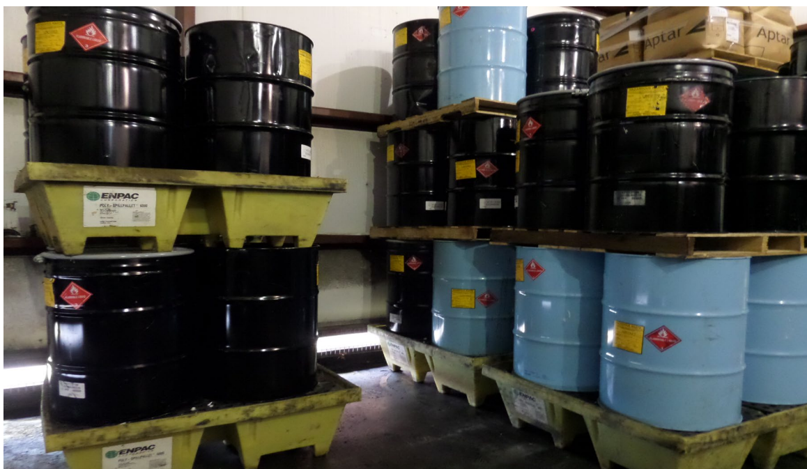
ITW Pro Brands. 90-Day or Less Accumulation Area. Inspectors observed 55-gallon containers accumulating hazardous waste in this area. Photograph 8 taken at 11:18 a.m.
