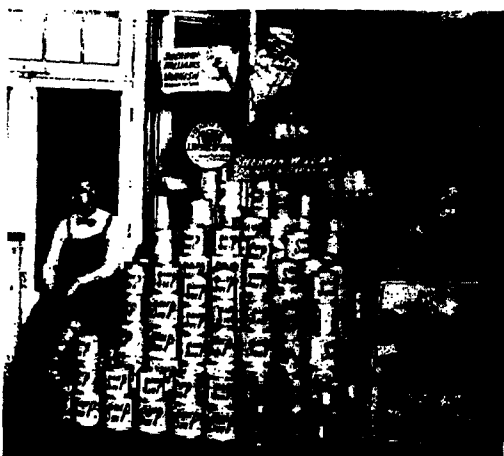
Our enterprising agents at Watertown, Wis., Schmutzler & Heisman, do the largest paint and wall-paper business in their section of the state. Mr. Walter Schlueter, store manager, shown in picture with his favorite line
