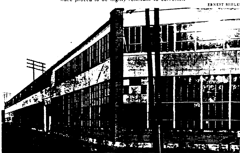
Lead coated corrugated steel sheets on this foundry building in Omaha, Nebraska, have proved to be highly resistant to corrosion
