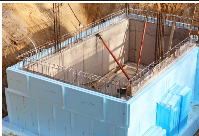
Figure 2.24 Extruded polystyrene foam boards for under grade (ground) construction
