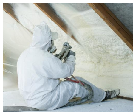
Figure 2.20 Spray foam Application
