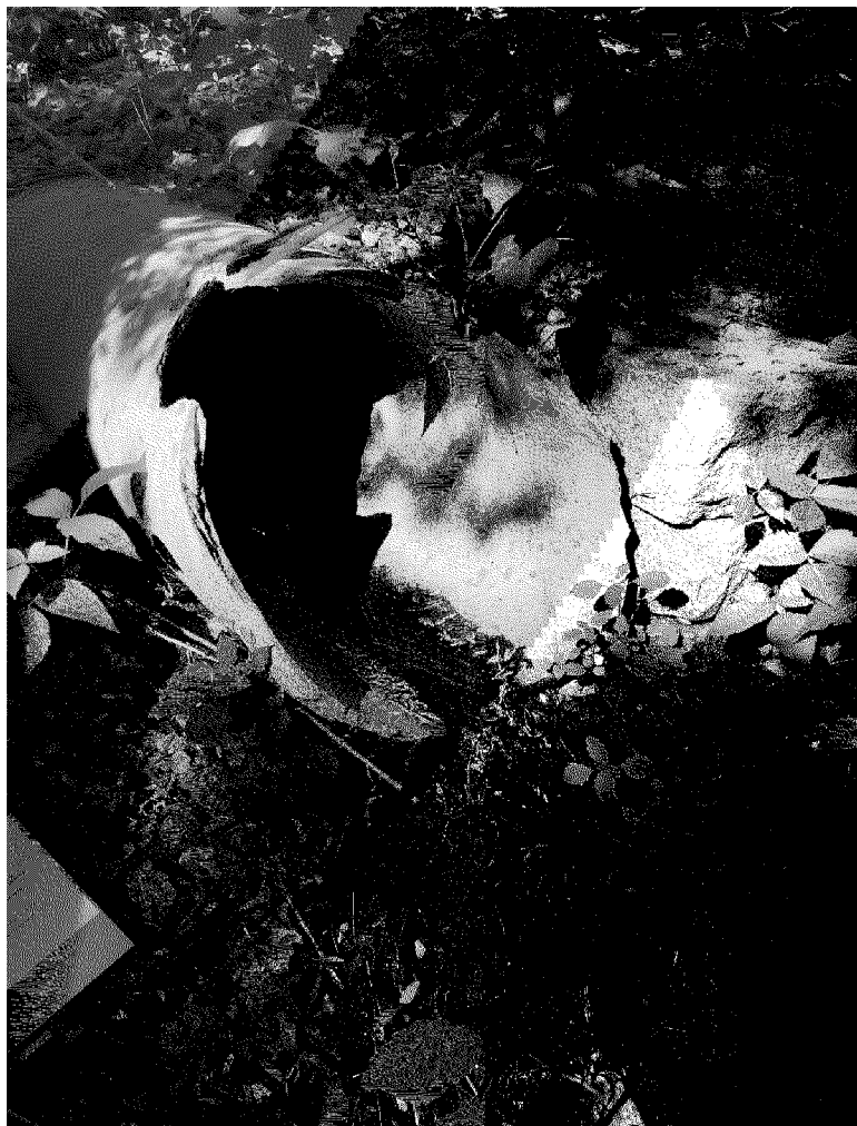
Renfrew (photo taken 5/24 at 08:48 AM): Outfall located on the northeast side of the Renfrew Street bridge over Bare Meadow Brook. Sample point is indicated by a red arrow.
