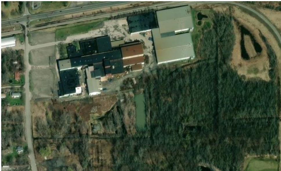
(Image displaying aerial view from Google Earth)
