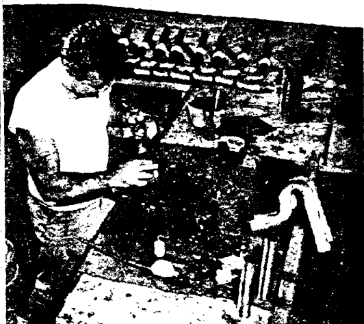
Traps and bend are wiped by experts and then . . .
