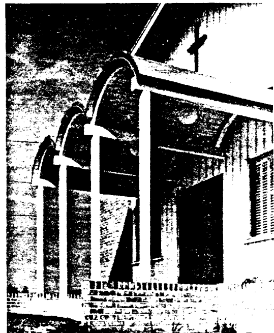
St. Luke's Wedding Chapel at the Naval Academy, Annapolis. Terne is used here for the barrel vaulted roof. Architects: Rogers, Taliaferro and Lamb, of Baltimore.
