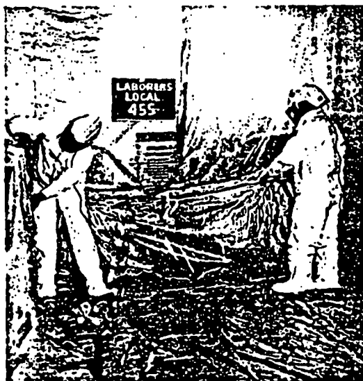
Steward Curt Jones, (l.), Laborers' Local No. 455, West Haven, Connecticut, and his brother member Lewis Cascagna, prepare the area prior to encapsulation.
