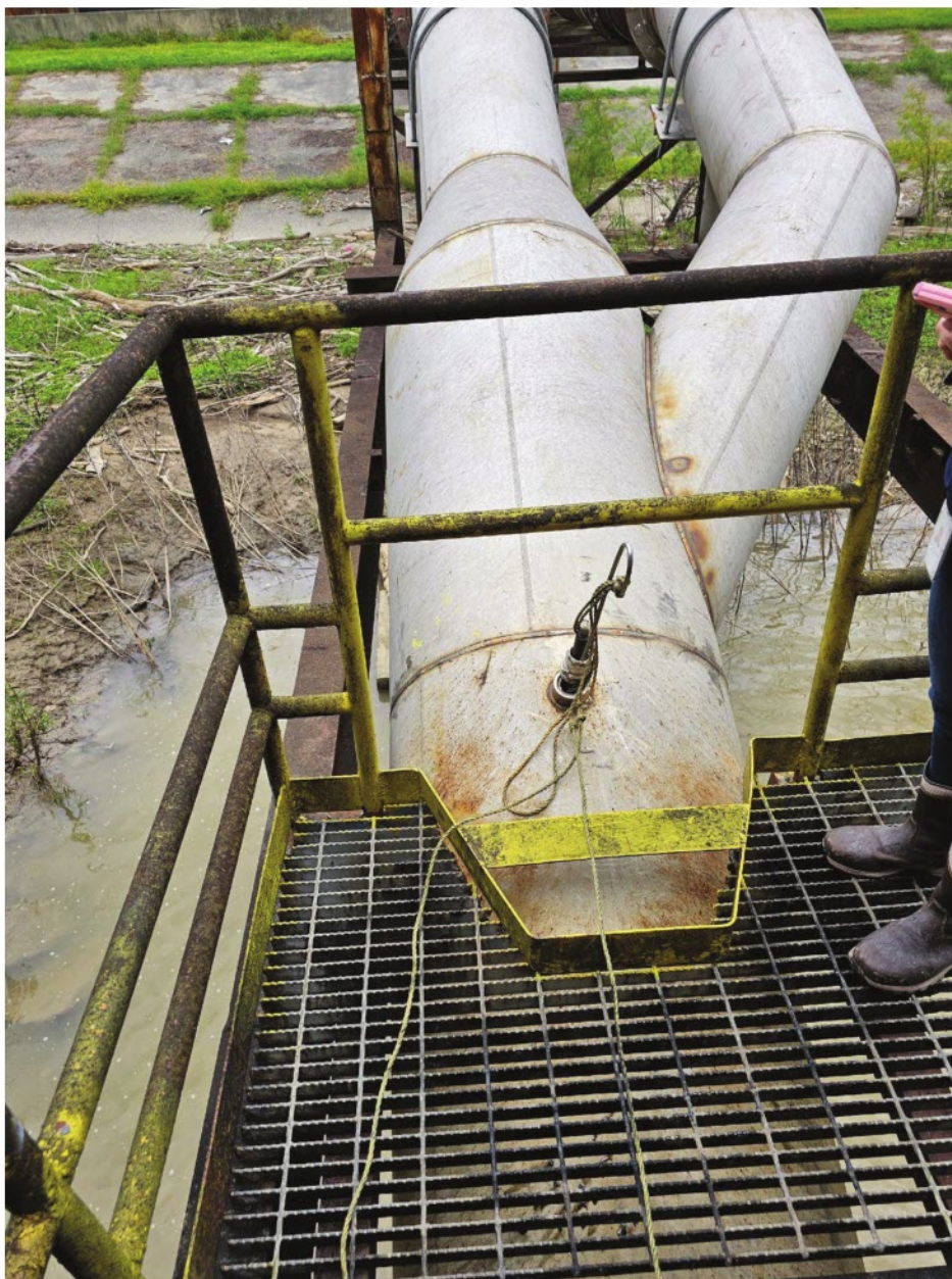
Outfall 001 Sampling Point. Outfall discharge is submerged.
