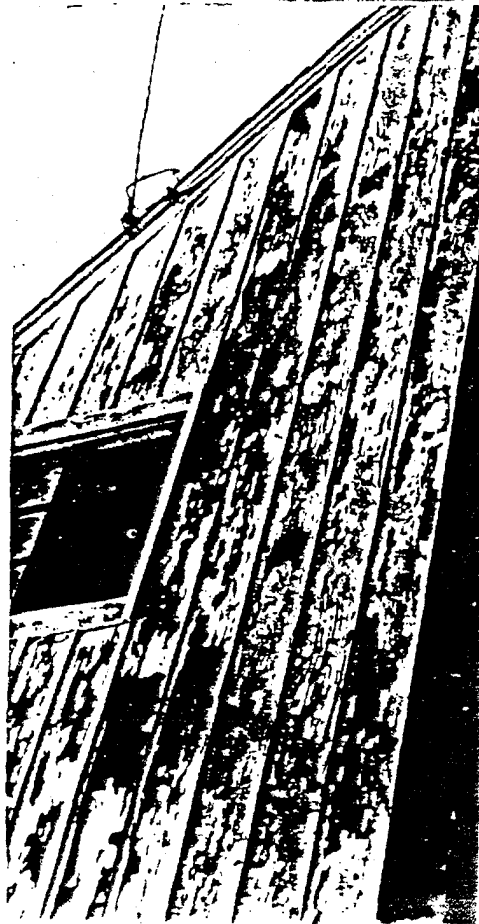
This paint is doing its best to save the painter the work of removing it. That which doesn't peel off will have to be forcibly removed, however, and the surface treated as new work.
