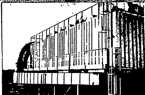
Series 12 baghouse controlling fume on induction furnace.
