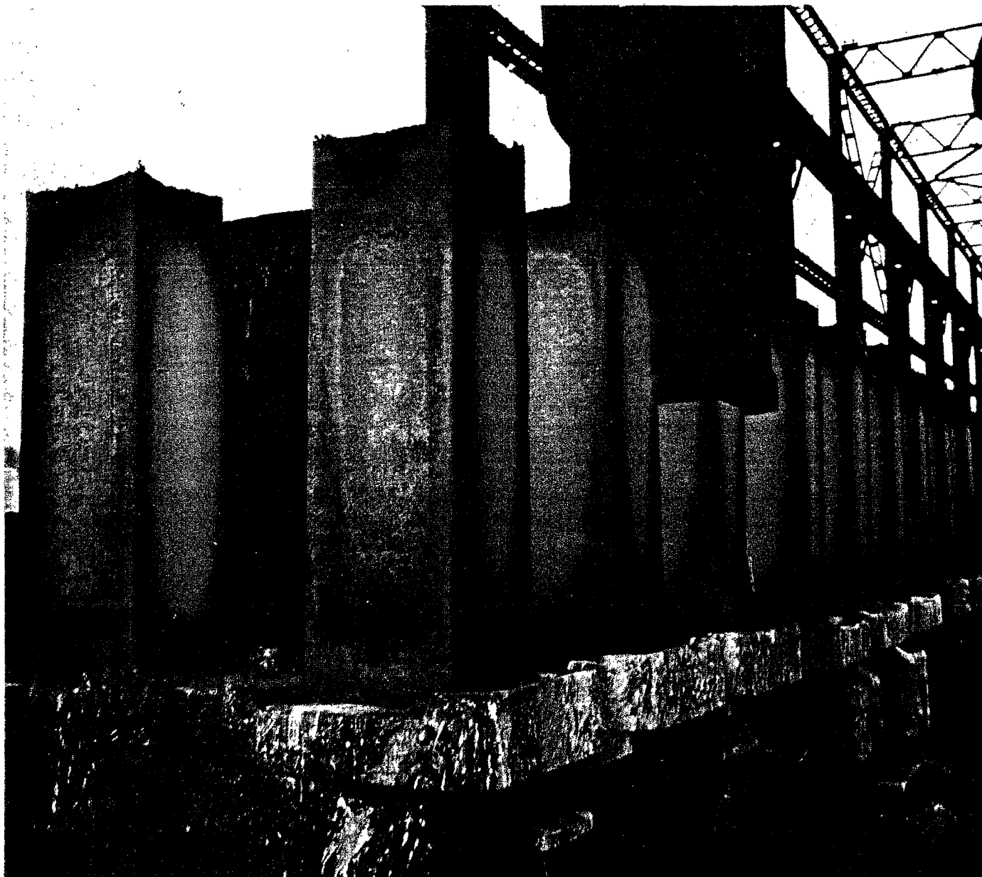
Removing molds (stripping) from hot Open Hearth ingots at the Lowellville, Ohio, Works of the Sharon Steel Corporation.
