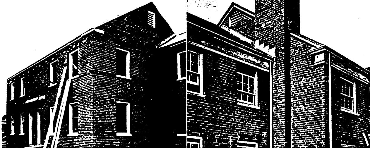
Below, cap flashings at roofs and cornice returns are built into brickwork.
