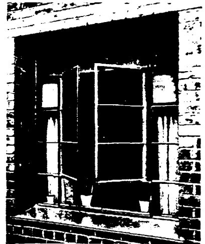
Detail of window sash sill and lintel with fresh coat of rust inhibiting red lead paint.
