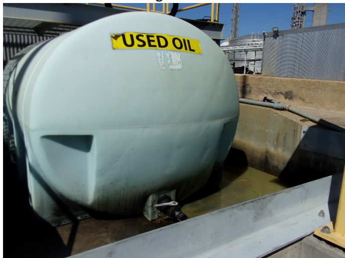
Photo-7 Oily Residue in Secondary Containment
