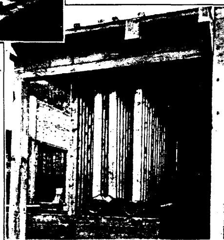
Top of elliptical hard lead pipes in gas cooler unit, showing water seal lead jackets.
