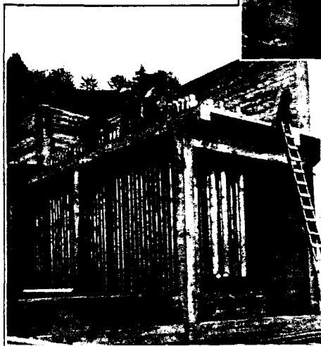
Top of elliptical hard lead pipes in gas cooler unit, showing water seal lead jackets.
