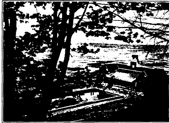
Swimming pavilion, Three Tree Point, Seattle, Wash., with Puget Sound in the background. E. J. Ivey, Seattle, architect.
