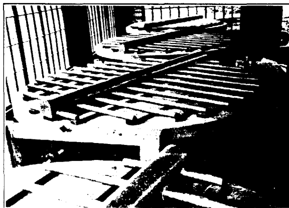
Lead piping in acid filter system tank bottoms. Tank walls were built on later.
