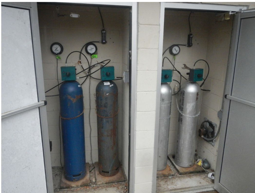
Figure 8: Chlorine (left) and sulfur dioxide gas (right) storage structure.
