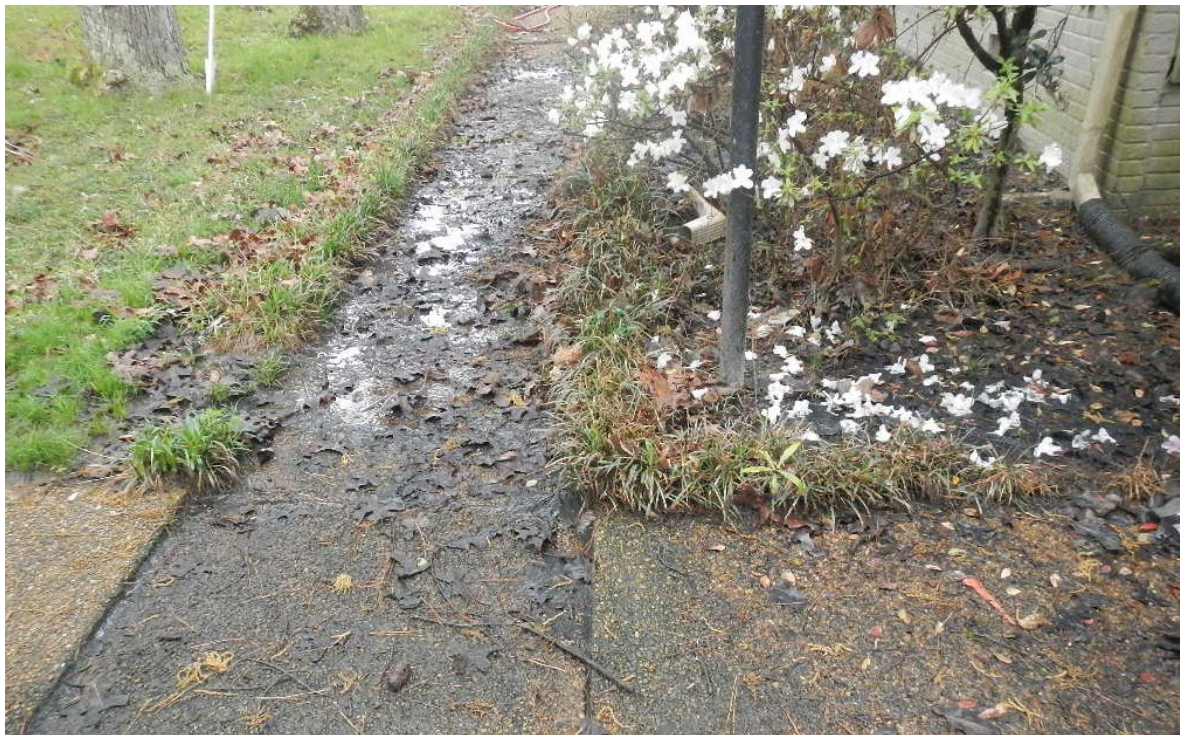
Photo 2. Raw sewage standing in the front walkway.
