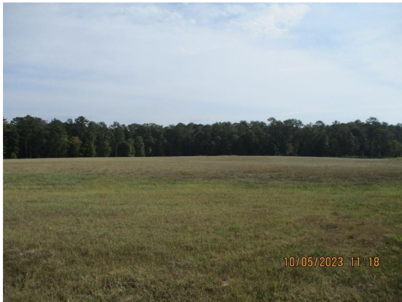
PHOTO # 8 – General view of capped Landfill C
