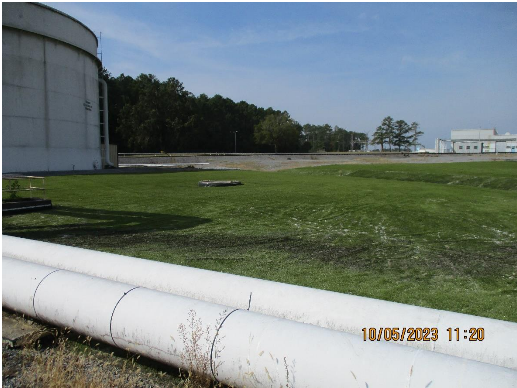
PHOTO #9 – General view of capped Landfill B
