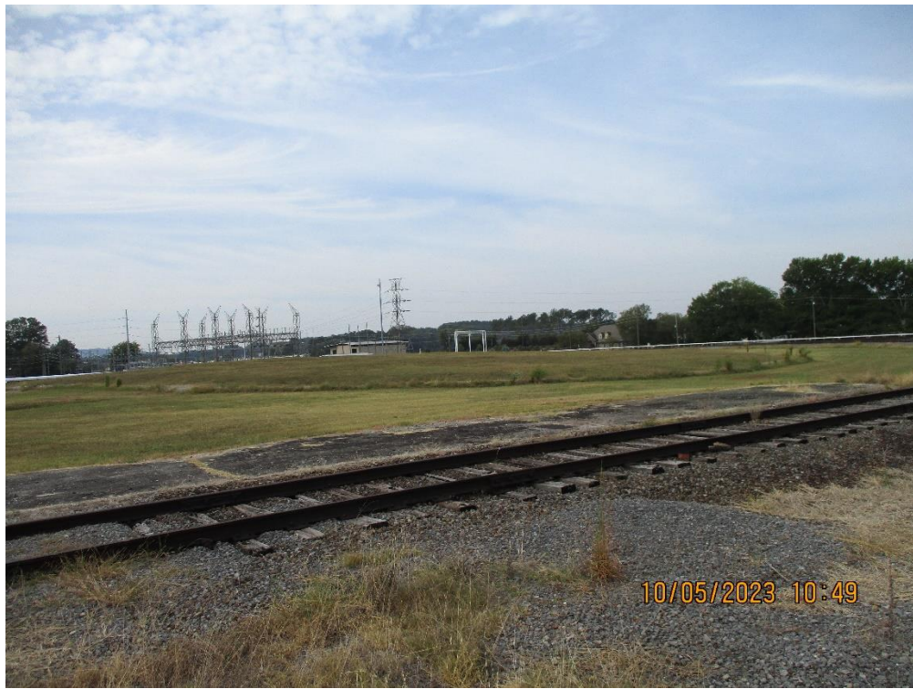
PHOTO #7 – General view of capped Landfill A
