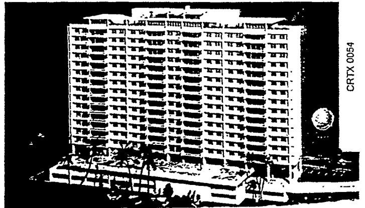
Fine plumbing fixtures by Crane are installed in apartments, housing projects, offices, factories and public buildings around the world. These new apartments are in Puerto Rico.
