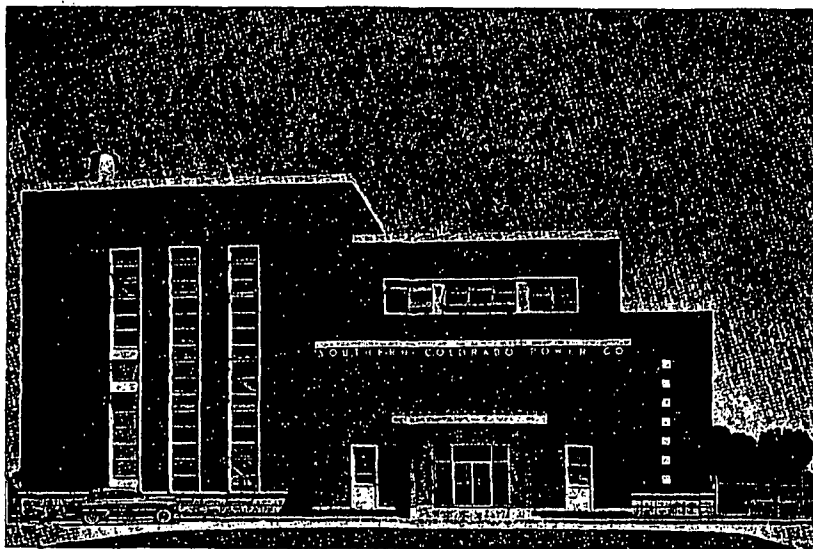
CLEAN LINES, modern look of today's power stations, even reflect sound engineering. But here's a plea for the same the smaller ones like this 7500-kw Rocky Ford, Colo. plant, attention to detail for the station's cooling-water service
