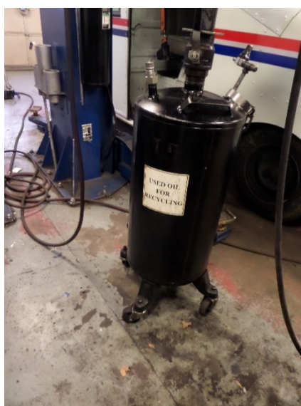
Picture 2: Used Oil Container on Skids, VMF
