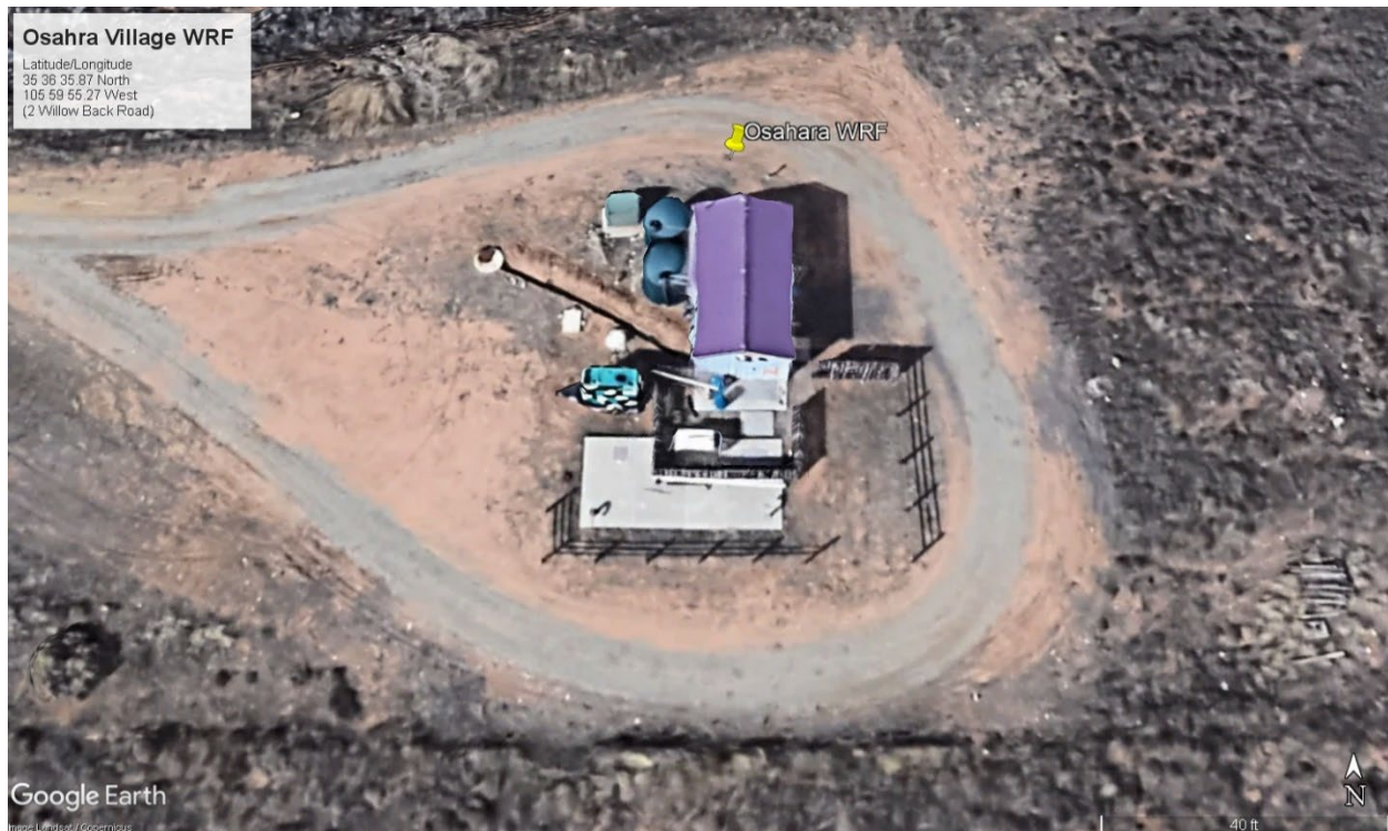
Aerial Image #1: Overall view of the Oshara Village Water Reclamation Facility location. Aerial from Google Earth Maps.
