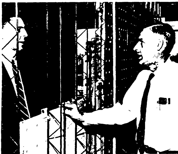
PLASTERING CONTRACTOR Charles J. Knight (right) explains time-and-money saving effected (in conduit installation and chase walls) on Trinity Tower job to U.S.G. Salesman Jim Sauter. For sound-comfort (46 db), units are isolated with 3¼-in. TRUSSTEEL stud party and corridor walls, finished one side with TR-1 resilient clips, ROCKLATH plaster base and plaster; opposite side is conventional wall of ROCKLATH and ¾-in. sanded RED TOP plaster.
