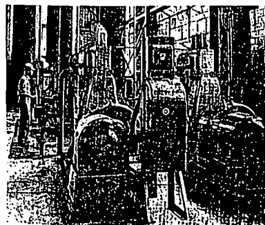
HYDRAULIC pumps and the accumulator in the background maintain 3000-psi pressure for molding presses. Smaller pumps in background serve the 500-psi system
