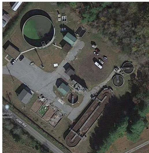
Figure 1: Aerial Display of the STP
