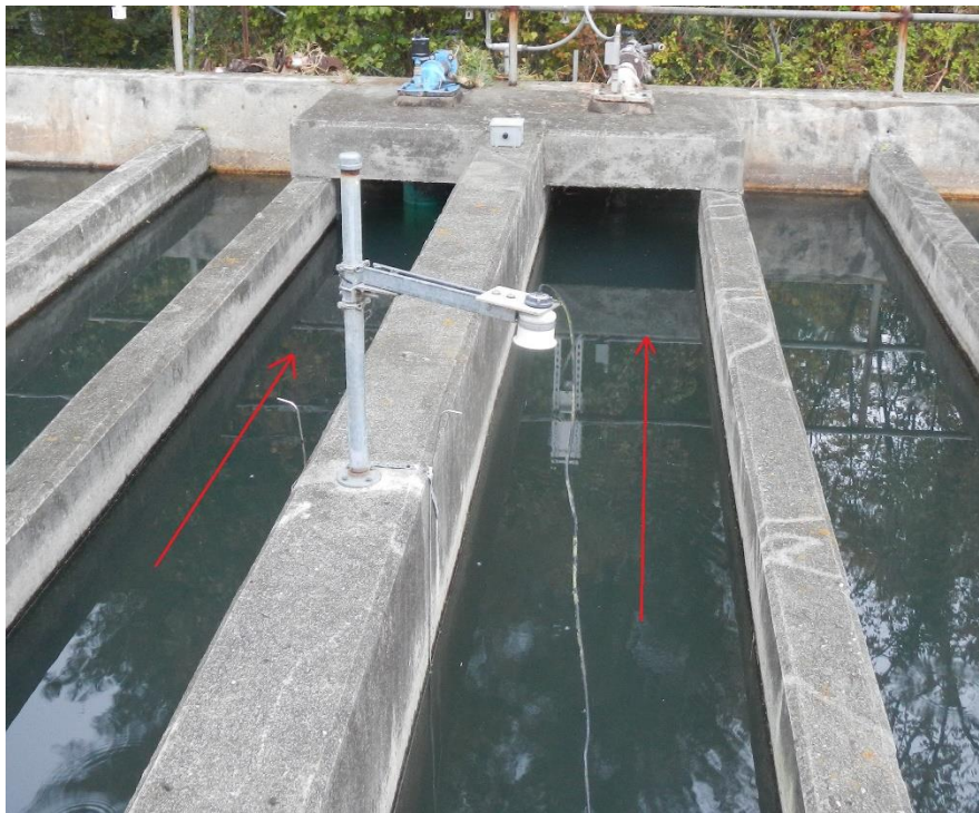
Figure 2. Effluent ultrasonic transducer. Red arrows represent separate Flow paths in the CCC.
