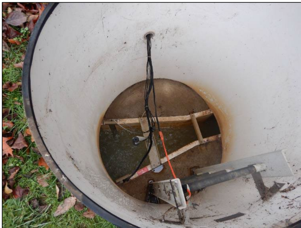
Photograph 28. (DSCN00090) View of the effluent flume for Outlet 011.
