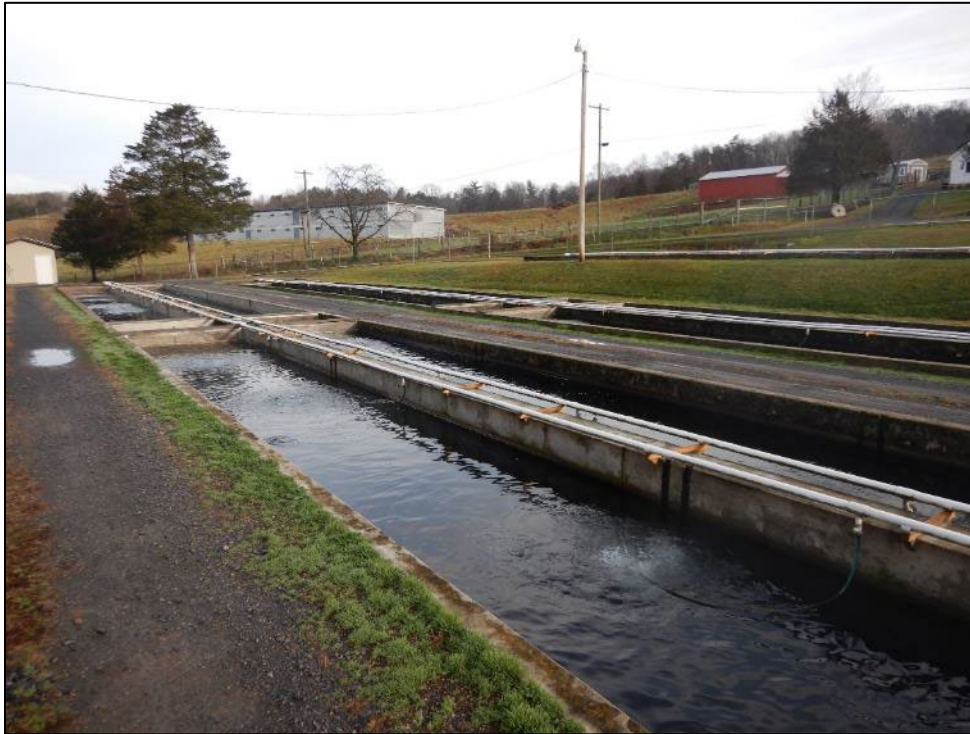
Photograph 7. (DSCN0044). View of the middle raceways.
