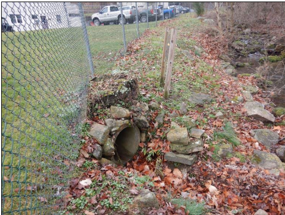
Photograph 30. (DSCN0124) View of the Outlet 009 pipe.
