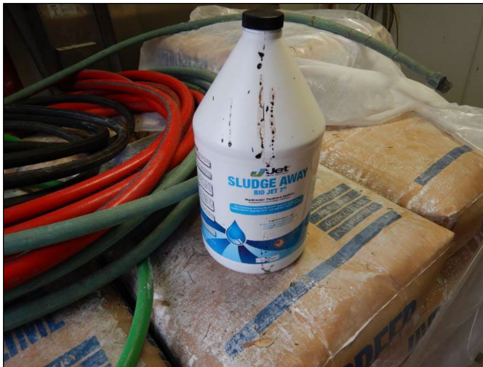
Photograph 24. (DSCN0079) View of the enzyme the Permittee was considering using inside the sludge holding tank. The label states the product is “Sludge Away Bio Jet 7®”. It is a “wastewater treatment additive” for residential, commercial, and municipal applications and is a “solution of non-toxic bacteria designed to enhance biological activity”
