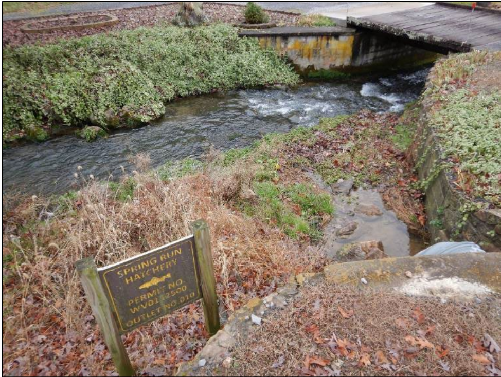
Photograph 31. (DSCN0112) View of Outlet 010.
