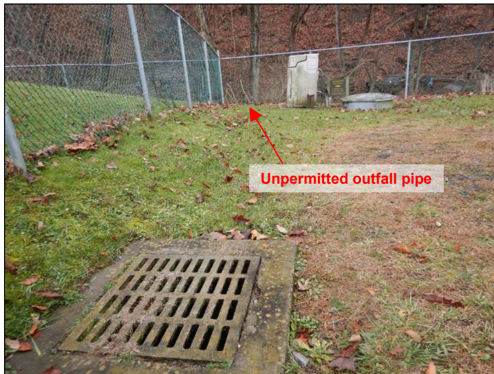
Photograph 35. (DSCN0096) View of the stormwater drain inlet upgradient of the unpermitted outfall pipe. The arrow call-out is pointing in the general location of the pipe.
