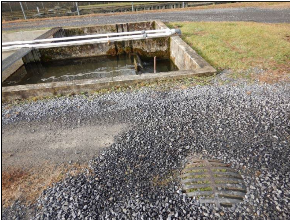
Photograph 40. (DSCN0120) View of a stormwater drain inlet between the middle raceways. Facility representatives stated that the stormwater drain inlets between the upper and middle raceways drain the infrastructure that conveys aquaculture wastewater to Outlet 011.
