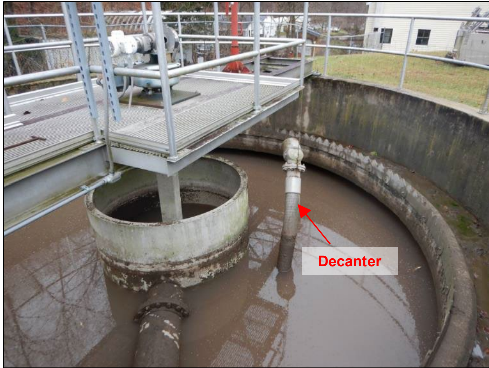
Photograph 13. (DSCN0066) View inside the clarifier. A decanter is used to discharge from the clarifier to Outlet 011.
