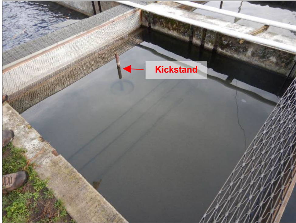
Photograph 9. (DSCN0047). View of one of quiescent zones in the middle raceways. The “kickstand” in the quiescent zone is removed during cleaning, thereby allowing the water to drain to the clarifier.
