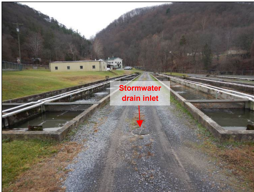
Photograph 38. (DSCN0119) View of a stormwater drain inlet between the upper raceways. Facility representatives stated that the stormwater drain inlets between the upper and middle raceways drain the infrastructure that conveys aquaculture wastewater to Outlet 011.
