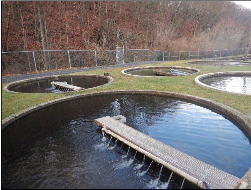
Photograph 1. (DSCN0031) View of the holding pools. Water that passes through these pools is discharged untreated to Spring Run via Outlet 008.
