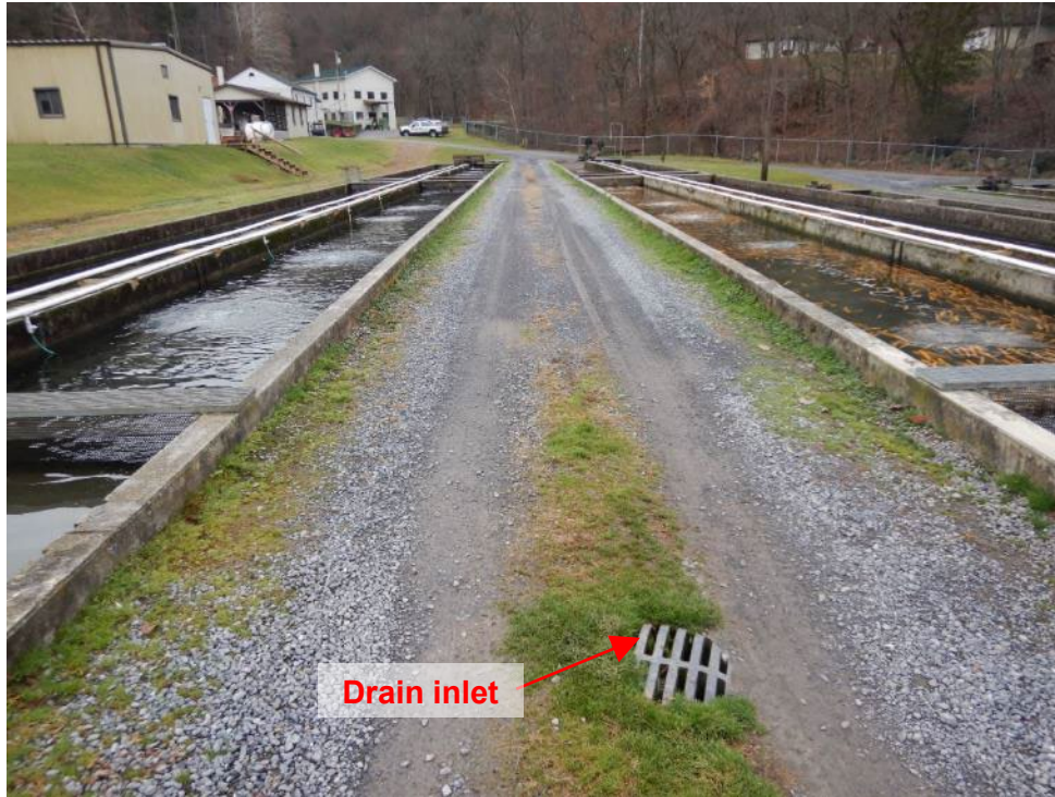
Photograph 39. (DSCN0121) View of a stormwater drain inlet between the upper raceways. Facility representatives stated that the stormwater drain inlets between the upper and middle raceways drain the infrastructure that conveys aquaculture wastewater to Outlet 011.
