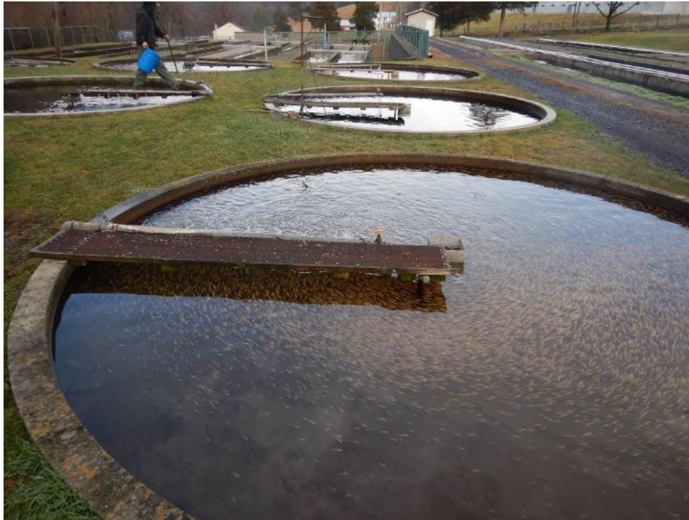
Photograph 3. (DSCN0035) View of the holding pools. Water that passes through these pools is discharged untreated to Spring Run via Outlet 008.
