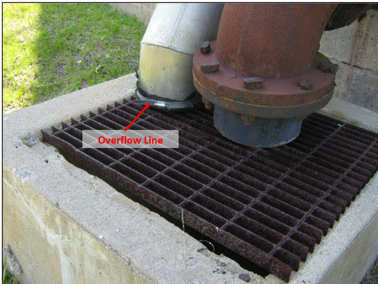
Photograph 48. Overflow Pipe, White Hall Tank #3 View of the terminus of the White Hall Tank #3 overflow pipe. The pipe was downturned, screened, and it terminated above a rectangular grate. Also visible in this image is a valved line that can be used to empty the tank.
