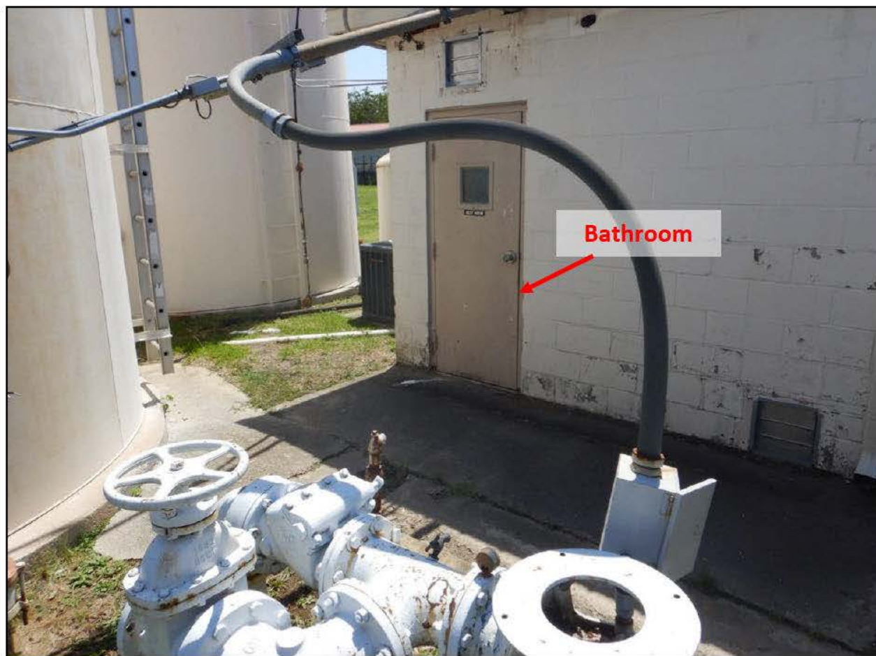
Photograph 40. Well No. 28 View of Well No. 28 and its proximity to a bathroom at White Hall WTP #4.
