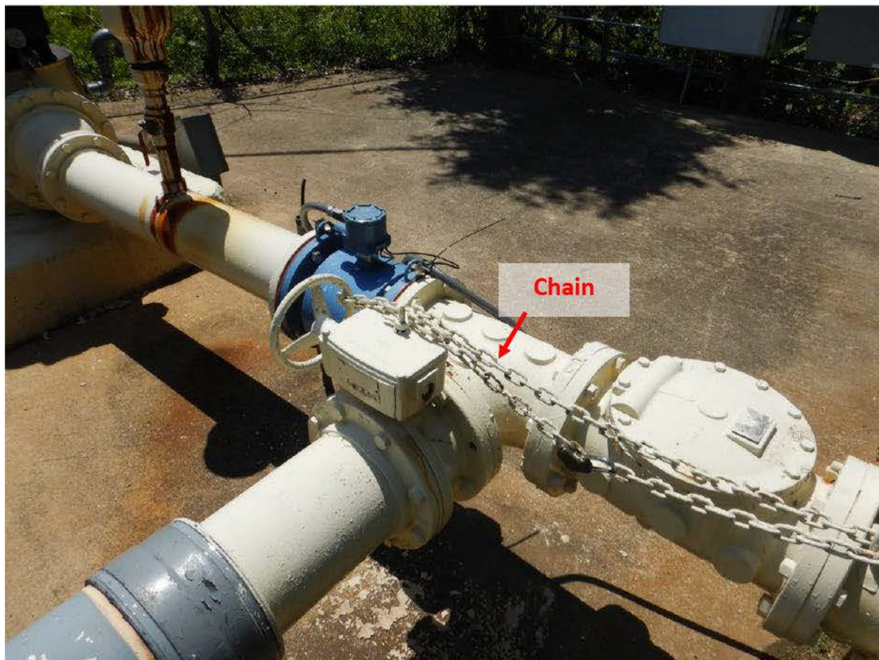
Photograph 17. Well No. 17 View of a chain that was threaded through the valve handle that was used to close the valve leading to the treatment system, as well as the handle to close the pump to waste line valve. The chain was in place to make sure the pump to waste valve did not get opened by mistake.
