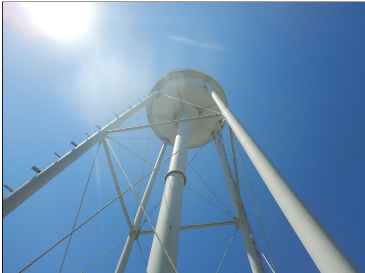
Photograph 42. White Hall Tank #1 View of the formally decommissioned, 50,000 gallon elevated White Hall Water Tank #1.
