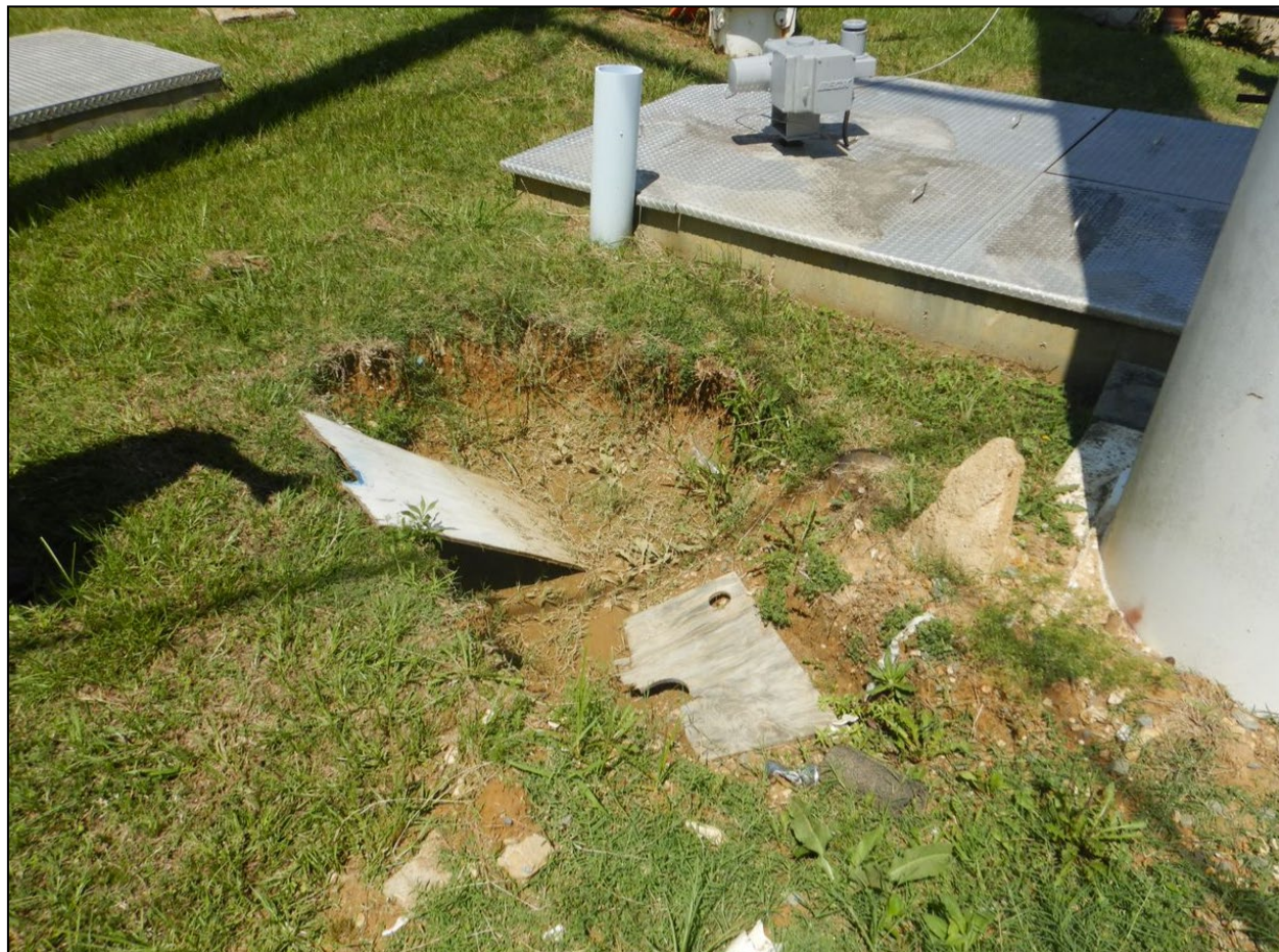
Photograph 43. Trench, White Hall Tank #1 View of the trench that was dug to formally cut and cap White Hall Tank #1 when it was formally decommissioned. The capped line was not visible.
