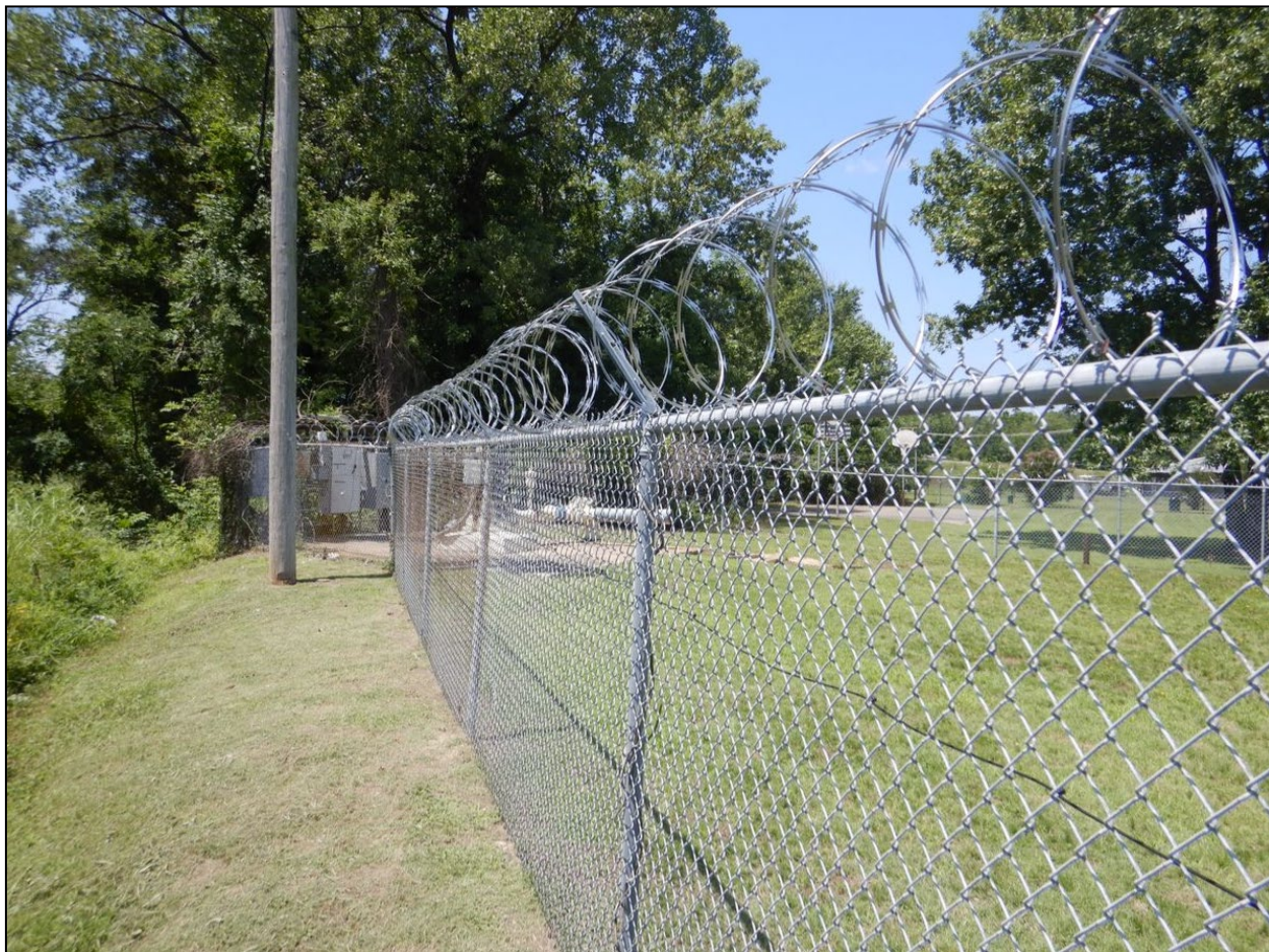
Photograph 13. Perimeter Fence, Well No. 17 View of the perimeter fence surrounding Well No. 17. The fence was locked and had razor wire.
