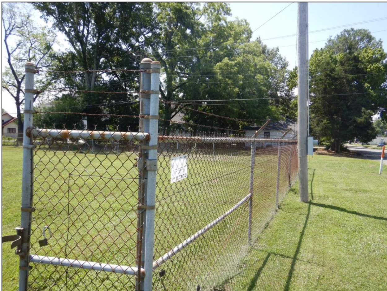
Photograph 7. Perimeter Fence, Well No. 18 View of the perimeter fence that surrounded Well No. 18. The fence was locked when the EPA Inspection Team arrived, and there was barbed wire.
