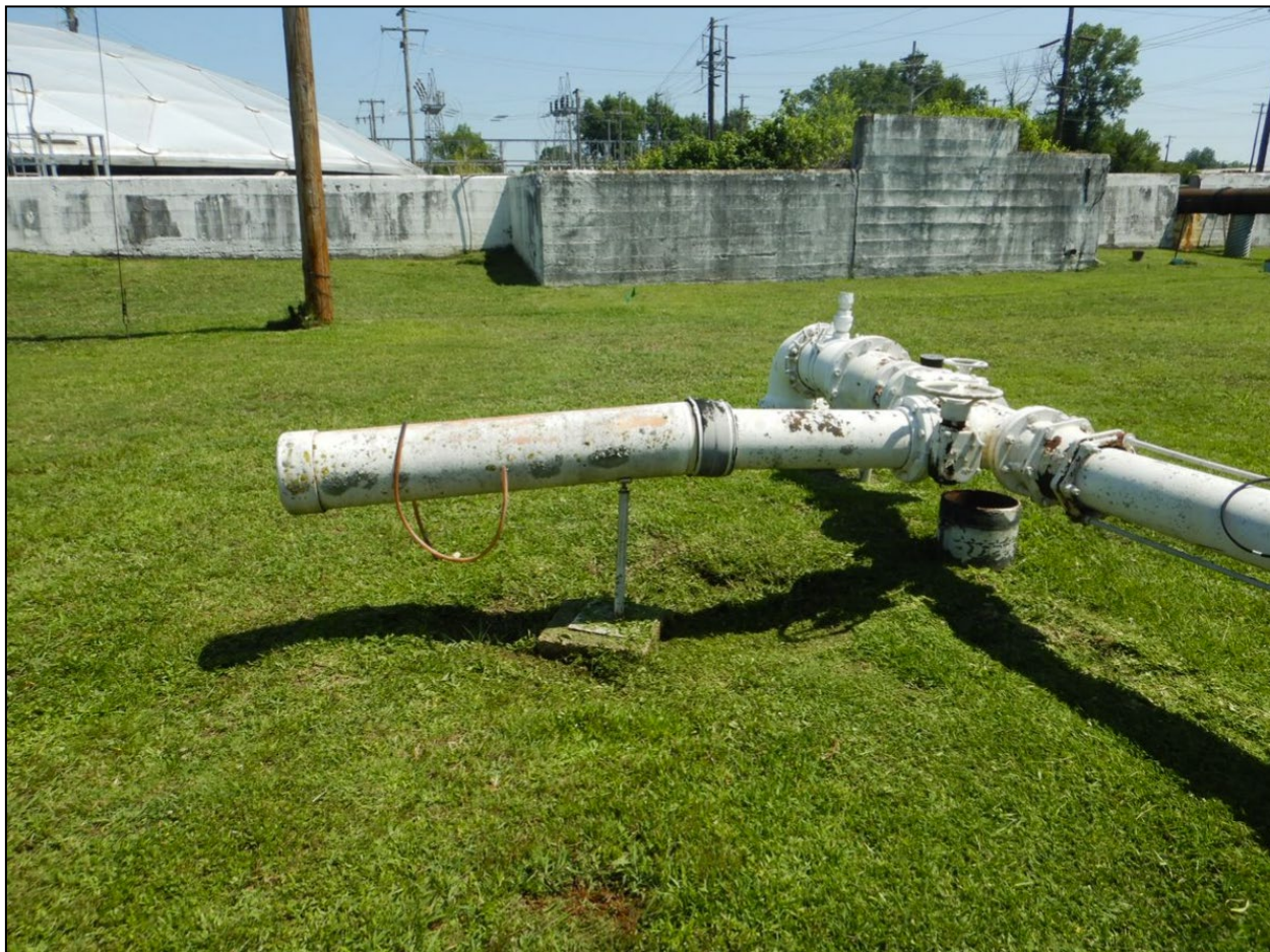
Photograph 1. Well No. 20 View of Well No. 20 that was inside fence line at the WTP #1 property. The well was functional at the time of the inspection and sending water to WTP#1 for treatment.
