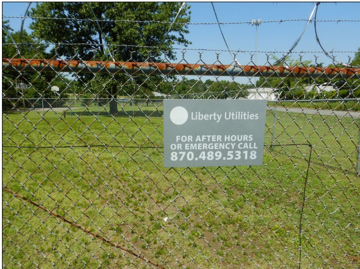
Photograph 14. Perimeter Fence, Well No. 17 View of a sign posted on the perimeter fence of Well No. 17 containing critical information about the System, including the System name and a number to call in case of an emergency.
