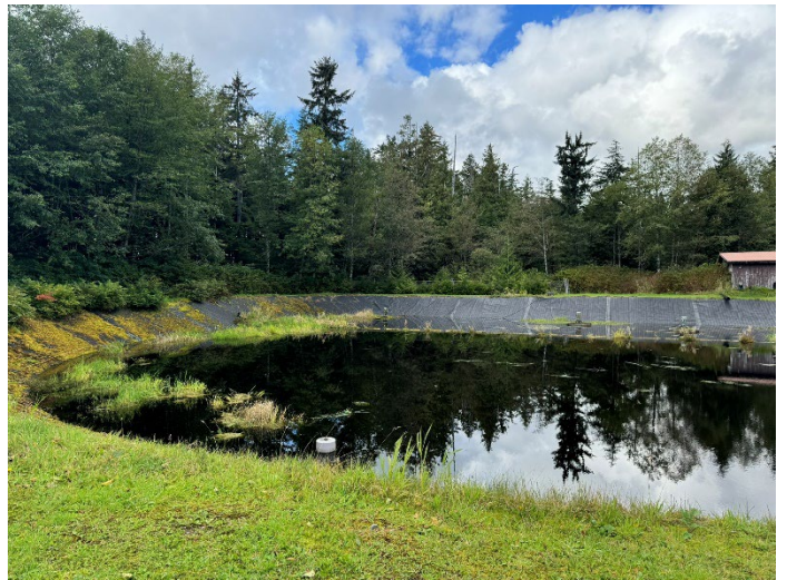
Photo #36 (8512) Description: Wastewater lagoon with vegetative growth.
