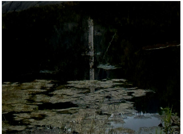
Photo #40 (8516) Description: Wastewater lagoon with vegetative growth.
