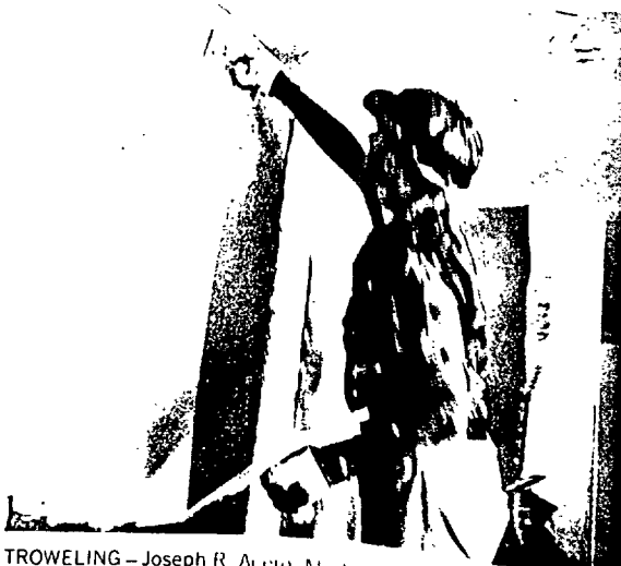
SMOOTH TROWELING—Joseph R. Acero, Martin Ruane's foreman, checks troweling consistency of IMPERIAL base coat. At 16 sq. yds. per hour with IMPERIAL finish, job includes colorant. Finish texture resembles simulated acoustical materials.
