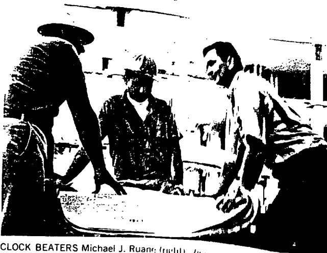
CLOCK BEATERS Michael J. Ruane (right), Joe Acero, president of Martin Ruane, Inc., Burlingame, and his foreman, Joseph R. Acero (center) plan schedule-beating strategy on next unit, with Pringle Construction Co.'s Job Superintendent John Dirnhofer. The $12.5 million complex will have 117 units with rents from $185 to $465.
