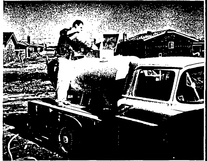
MOBILE UNIT'S 250-GAL. TANK is replenished at central storage location, eliminating need for stockpiling PERF-A-TAPE cement at various job sites.
