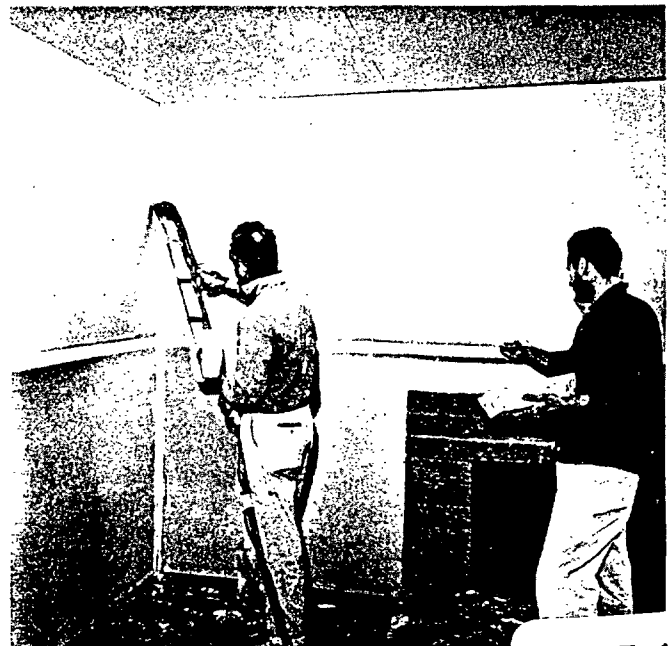
CONTINUOUS FLOW from hose (below) furnishes taper with cement while second member of team follows with hand tool.
