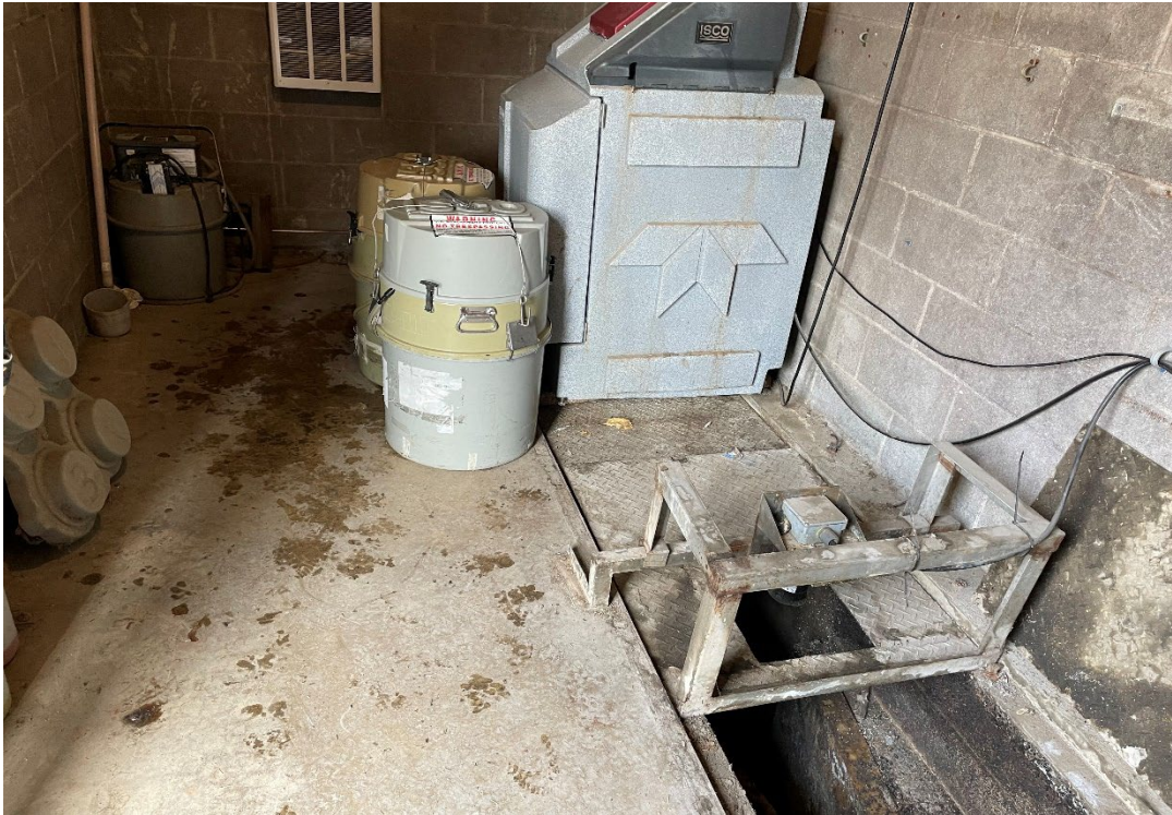
Photo #2. The collection tube to the facility's composite sampler was observed to be dirty.
