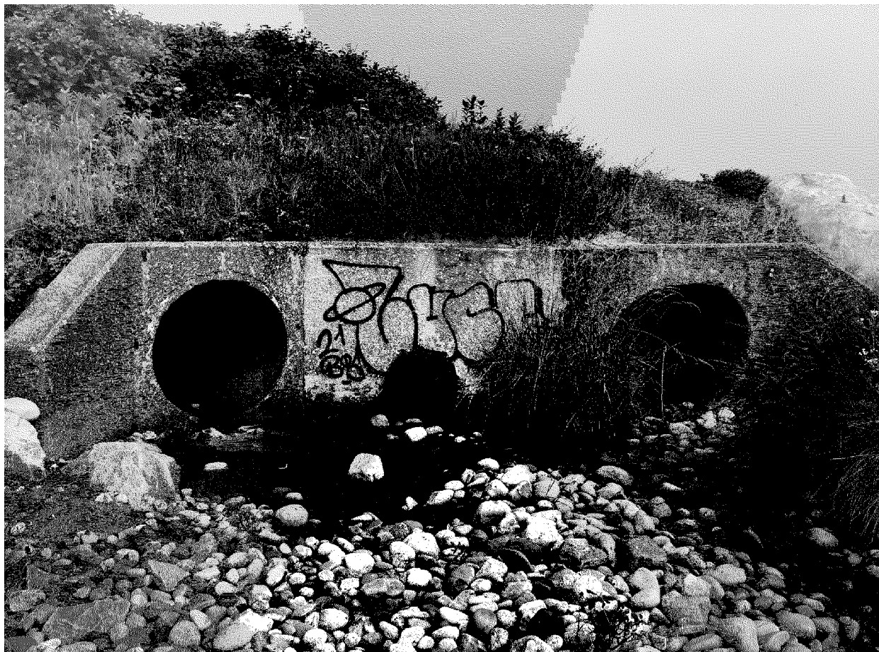
SB02 (left) & SB03 (right): Pair of reinforced concrete outfalls located at the southern end of Scarborough State Beach.
