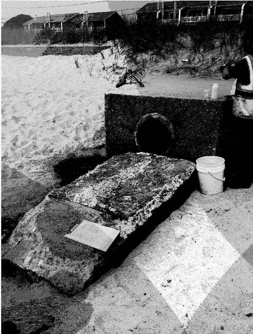
SB06: Reinforced concrete outfall located on Scarborough Beach across the street from Walcott Ave.
