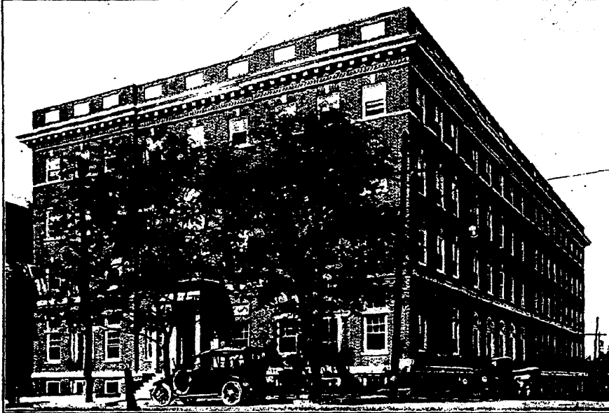
C. E. Kounts, of J. E. Ferguson & Co., Architect, Hagerstown, Md.
