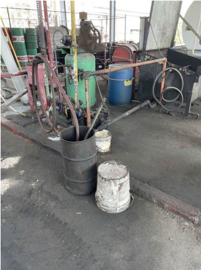
Photograph 18: Used oil container for pump operations that is not closed or labeled.
