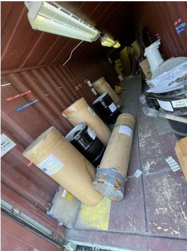
Photograph 30: Connex container for UW. Three UW lamp containers are not fully closed.
