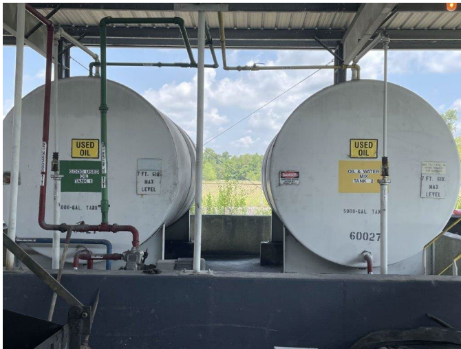
Photograph 17: Two 5,000-gallon used oil tanks that are labeled as used oil.
