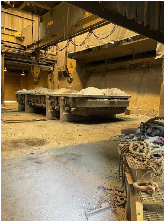
Photograph 32: Building 138, Pot repair and cleaning area.
