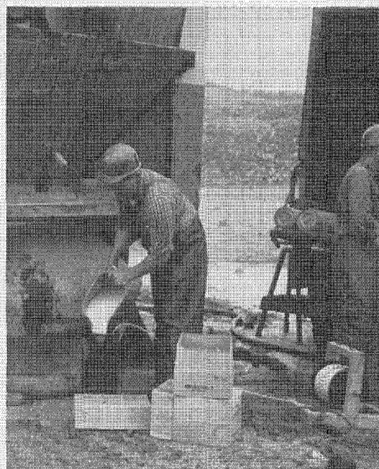
Crews pour free-running Pelletol 1 into 56-foot-deep holes to supplement main explosive.
