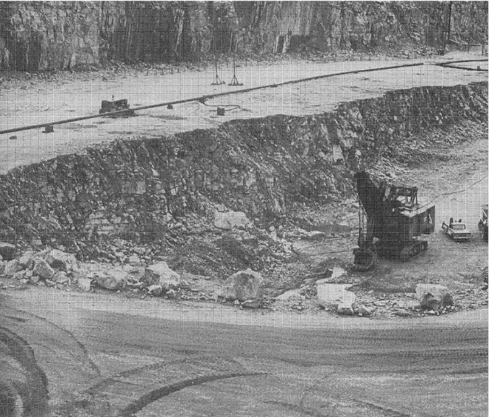
Big shovel digs fragmented rock in 4-million-cubic-foot hole blasted by one shot at J&L's open ore pit at Star Lake, N.Y.
