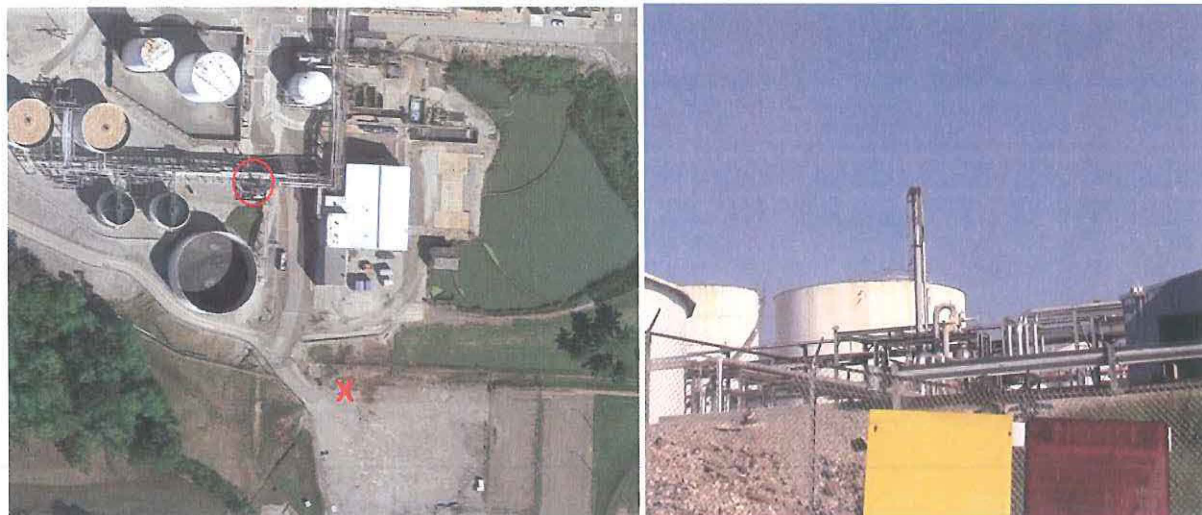
Figure 1. South flare. A steam assisted flare. Left: Google map with a red circle indicating the location of the flare and a red "X" indicating the location of the VISR instrument. Distance: 276 ft. Right: A photo of the flare taken during the test.
