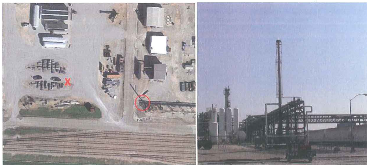
Figure 2. North flare. A steam assisted flare. Left: Google map with a red circle indicating the location of the flare and a red "X" indicating the location of the VISR instrument. Distance: 180 ft. Right: A photo of the flare taken during the test.
