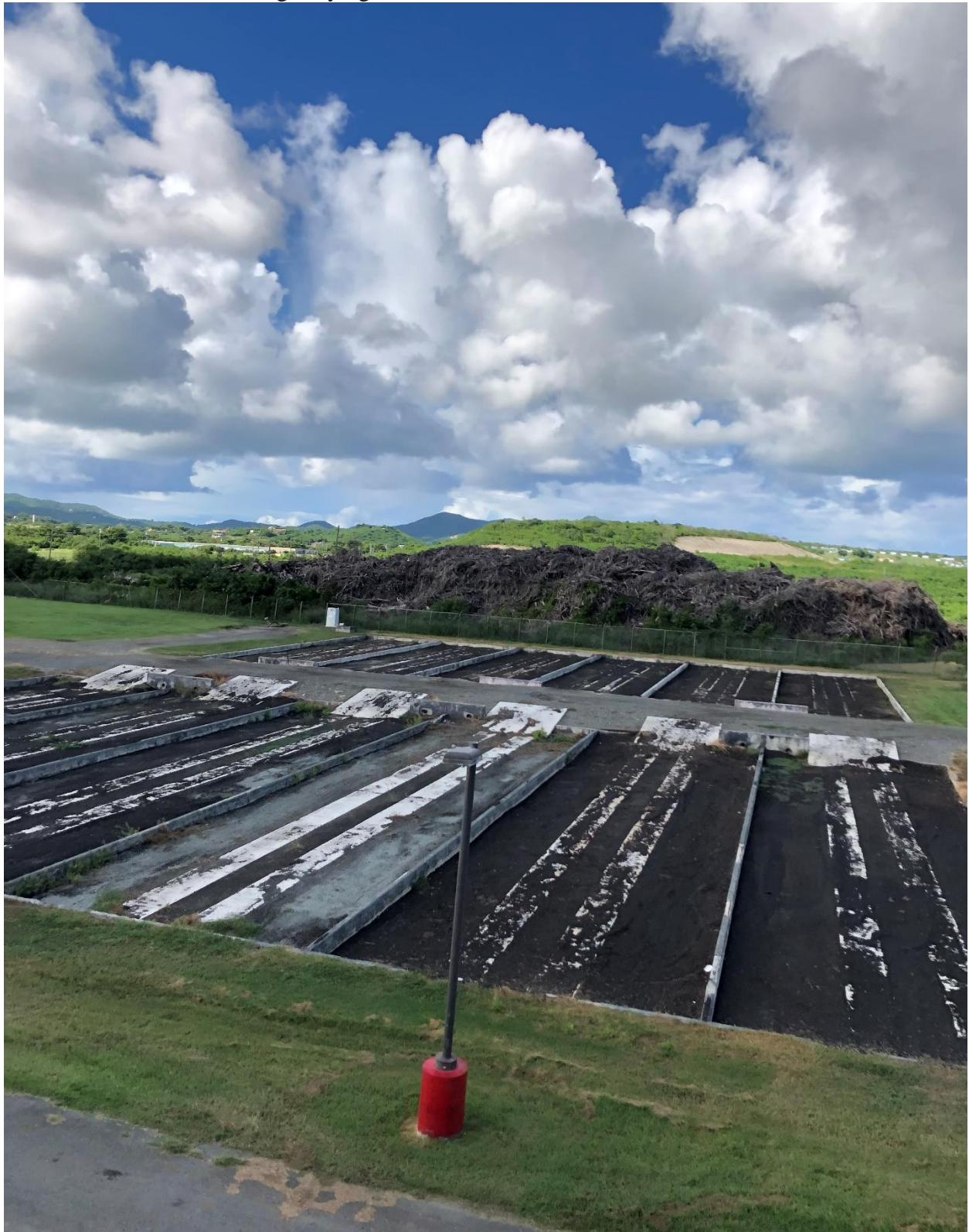
Photo #8: View of the sludge drying beds.
