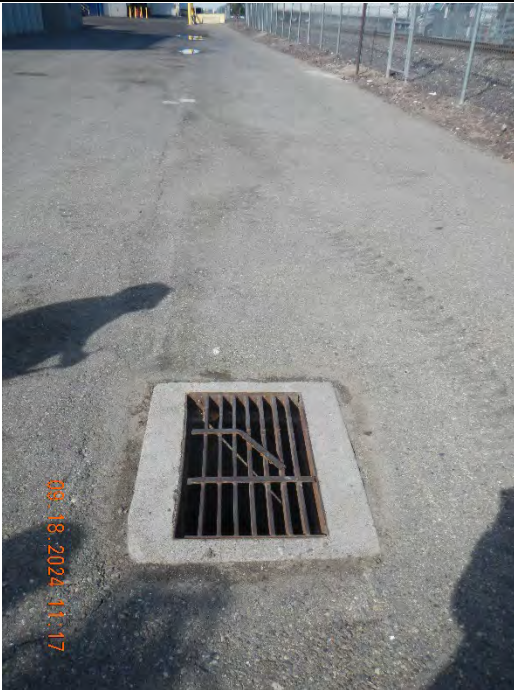
Photo #:03 (DSCN3910) Description: Facing west, photo of catch basin located south of the railroad.
