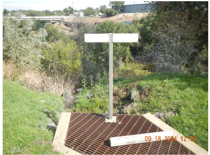
Photo #:18 (DSCN3925) Description: Facing east, photo of the Outfall 008 discharge location and grit chamber overflow discharge location Outfall 005.
