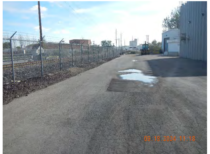
Photo #:04 (DSCN3911) Description: Facing east, photo of drainage area south of the railroad.
