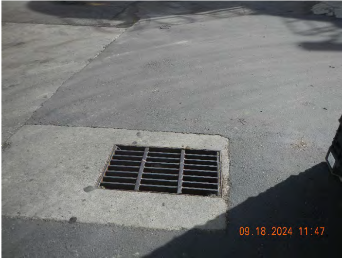
Photo #:17 (DSCN3924) Description: Photo of catch basin near the Hyster (forklift) maintenance shop.
