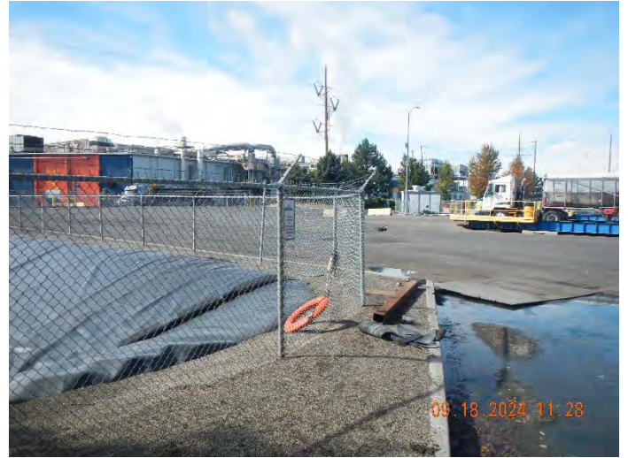
Photo #:10 (DSCN3917) Description: Facing southwest, photo of the north end of the stormwater system/pond.
