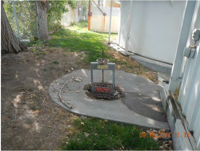
Photo #:01 (DSCN3908) Description: Facing south, photo of the decommissioned Outfall 002. The collection area is now routed to the main stormwater line, discharging to the collection pond.
