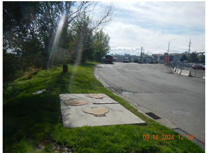
Photo #:20 (DSCN3927) Description: Photo of the oil/grit chamber/seperator associated with Outfall 005.
