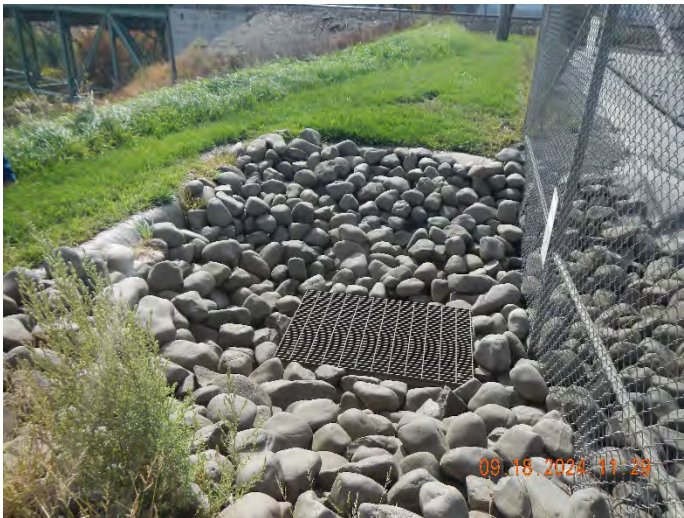
Photo #:11 (DSCN3918) Description: Facing south, photo of stormwater Outfall 003. Overflow of the stormwater collection system/pond.
