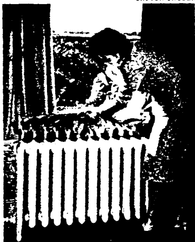
Placing lead foil reflective insulation behind radiator.
