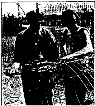
Cages being welded by Allan Portable Welding Machine
