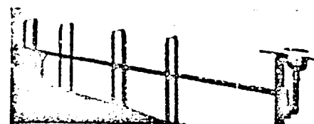
One of the vented waste lines from the lead cup sink at the U.S. Army Medical Depot at Fort Detrick, Md., showing the 2-in. trap seal.
