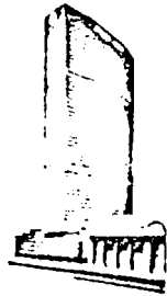
This 37-story New York skyscraper rests on lead-asbestos anti-vibration pads.
