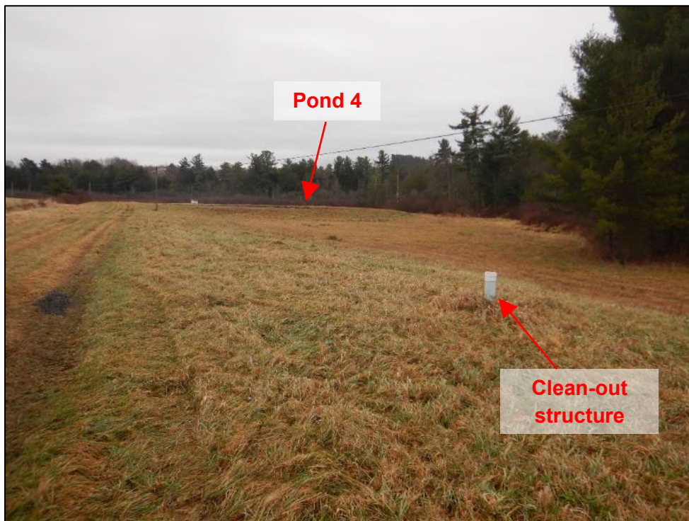
Photograph 12. (DSCN9108) View of what appeared to be a clean-out structure for the transfer pipe between Pond 3 and Pond 4.
