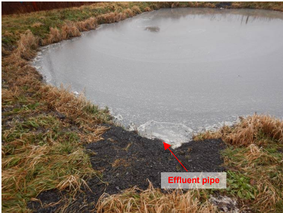
Photograph 4. (DSCN9094) View of effluent end of Pond 1.
