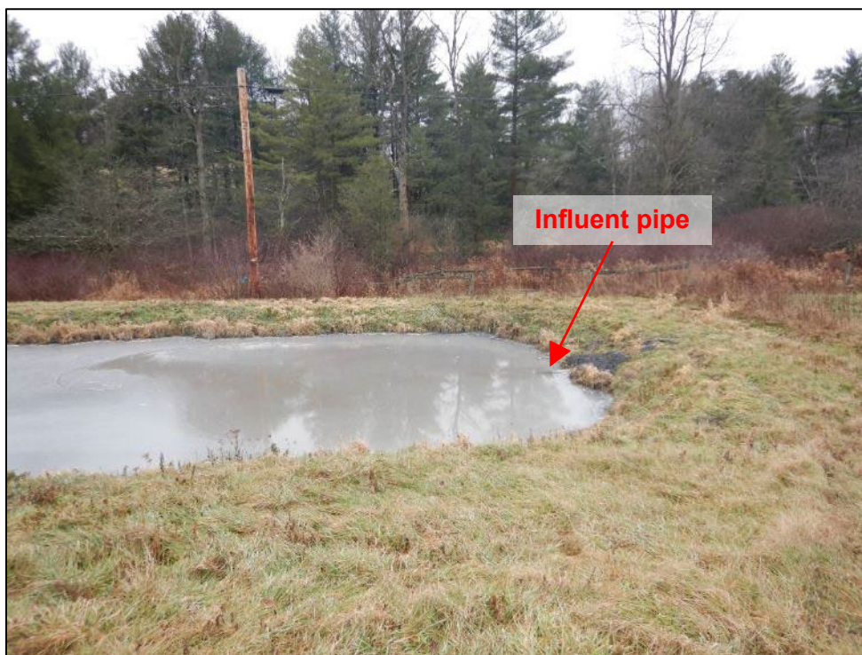
Photograph 2. (DSCN9092) View of influent side of Pond 1, which is on the western end of the pond.
