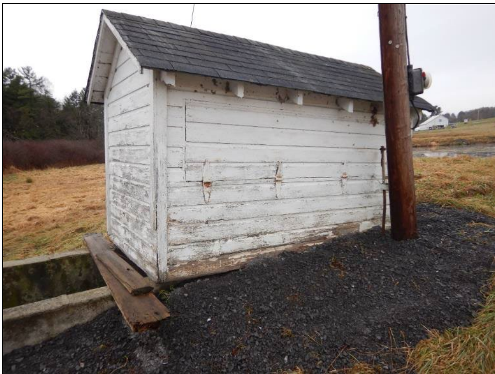
Photograph 24. (DSCN9120) View of shed after the effluent weir.
