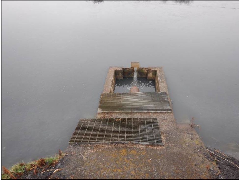
Photograph 17. (DSCN9115) View of effluent weir in Pond 5.
