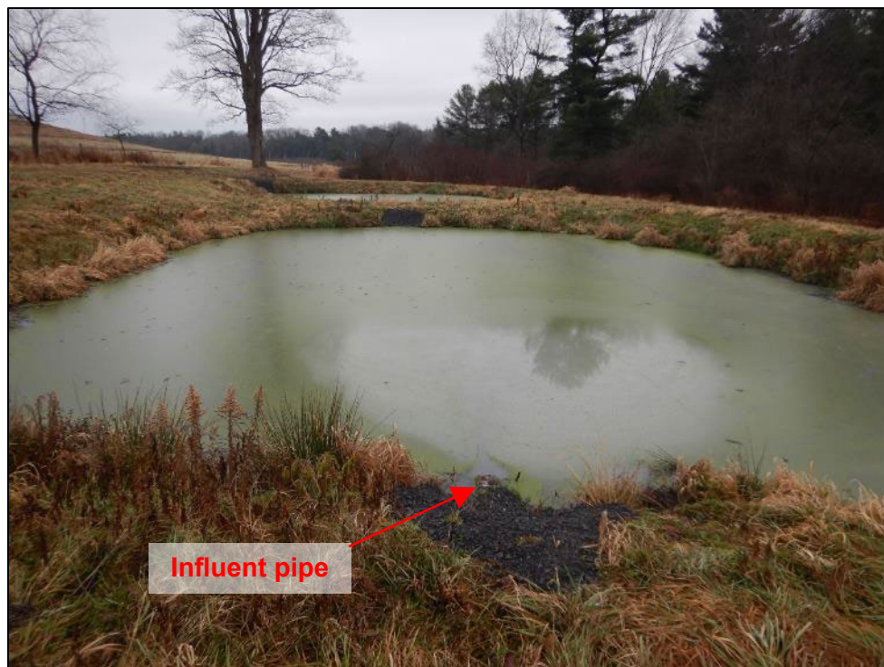
Photograph 6. (DSCN9098) View of Pond 2, facing east, from the influent end of the pond.
