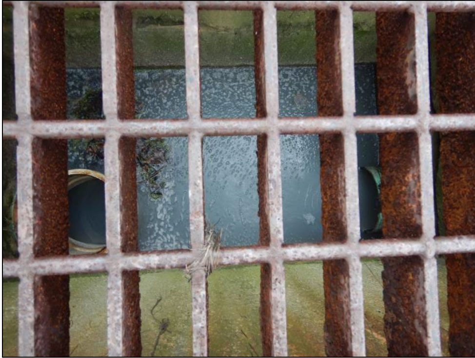
Photograph 11. (DSCN9107) View inside transfer structure in between Pond 3 to Pond 4.
