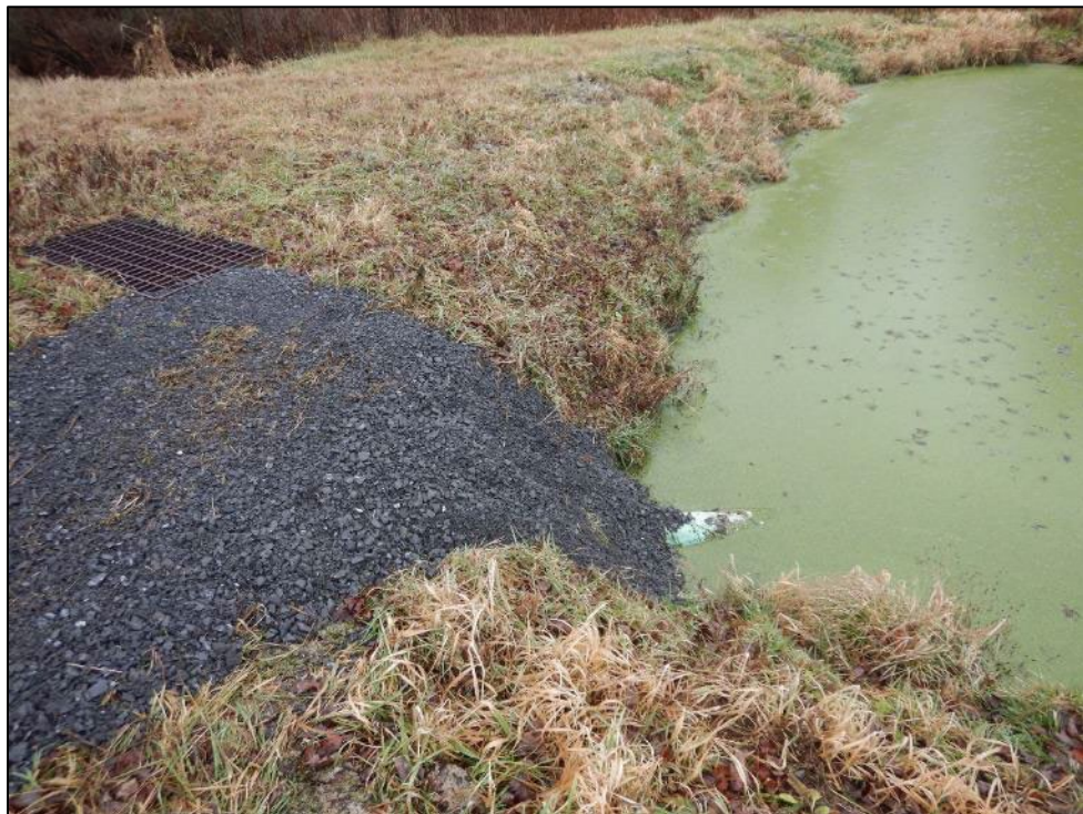
Photograph 10. (DSCN9104) View of effluent end of Pipe 3. Wastewater enters a transfer structure prior to flowing to Pond 4.
