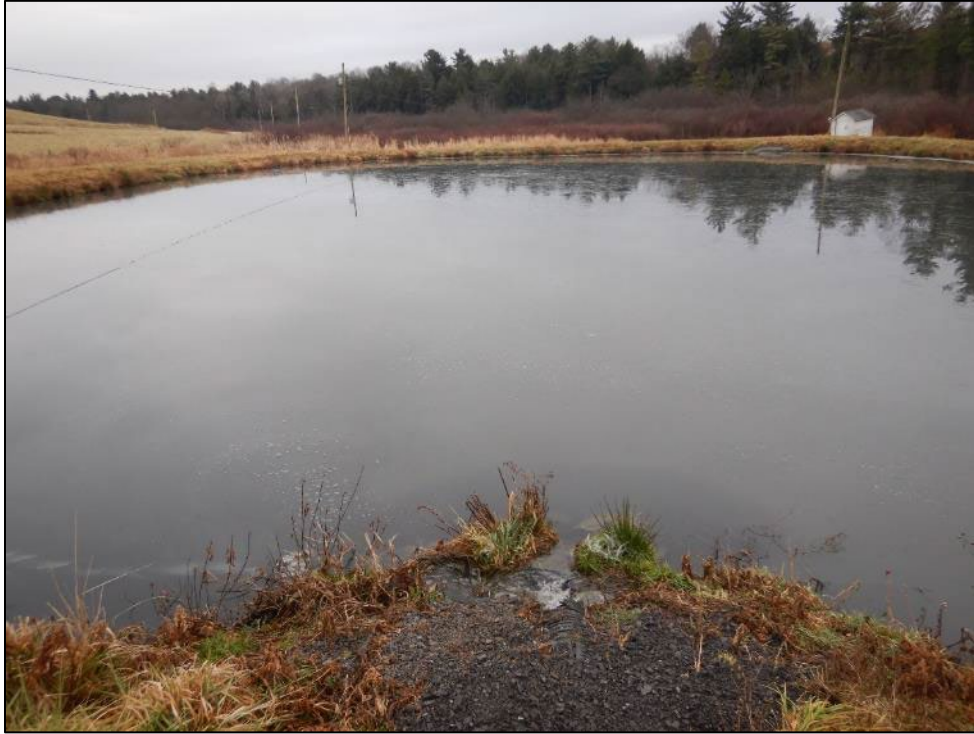
Photograph 15. (DSCN9114) View of Pond 5, facing east, from the influent end of the pond.
