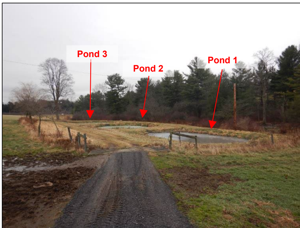
Photograph 1. (DSCN9091) View of Ponds 1, 2, and 3 from the access road.
