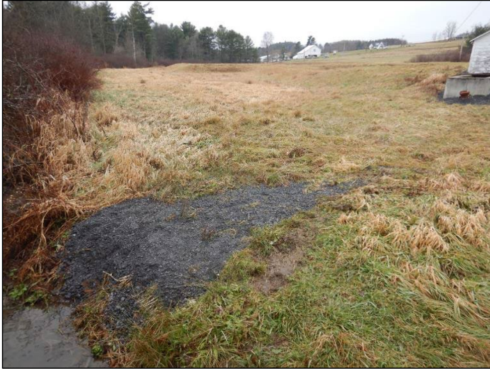
Photograph 21. (DSCN9124) View of Outlet 001 in relation to the chlorine contact tank.
