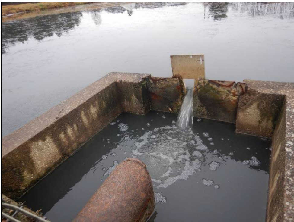
Photograph 18. (DSCN9116) View of effluent weir in Pond 5. The Permittee obtains flow measurements at this weir.
