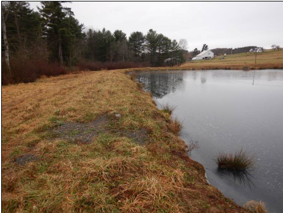
Photograph 16. (DSCN9133) View of Pond 5, facing northwest.
