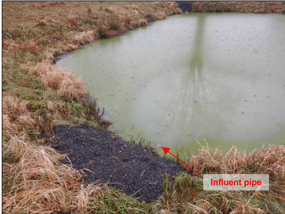
Photograph 9. (DSCN9103) View of the influent pipe for Pond 3.
