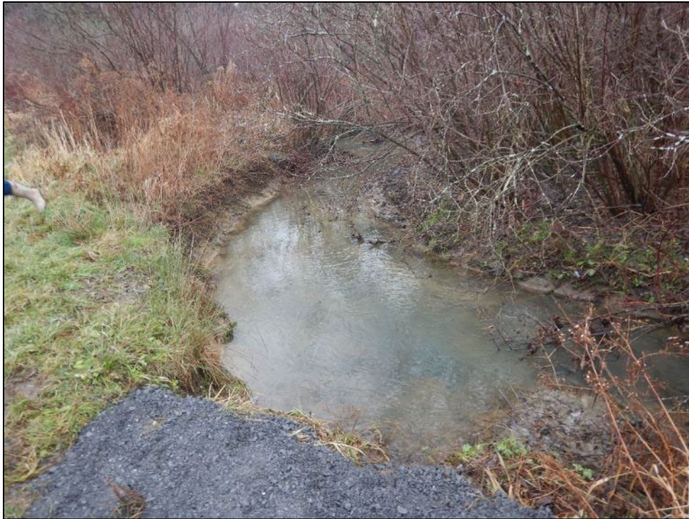
Photograph 23. (DSCN9127) View of Outlet 001, looking downstream of Outlet 001.
